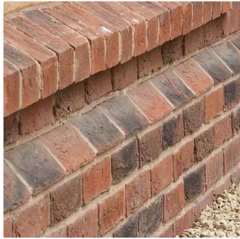
Brick Plinths & Detailing
