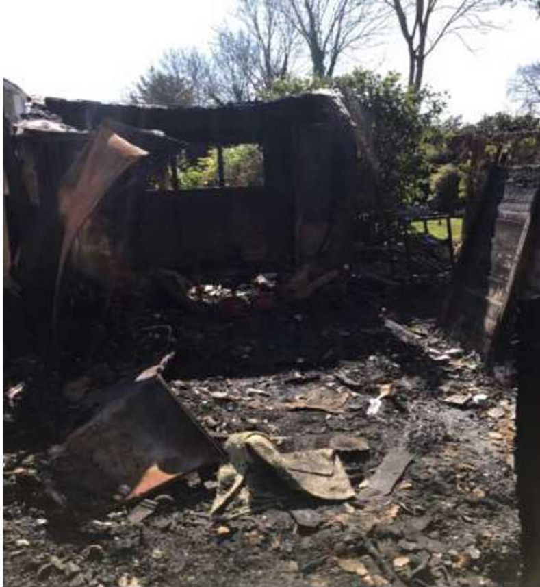
Photo 1 : Charred remains of pre-existing garden structure
