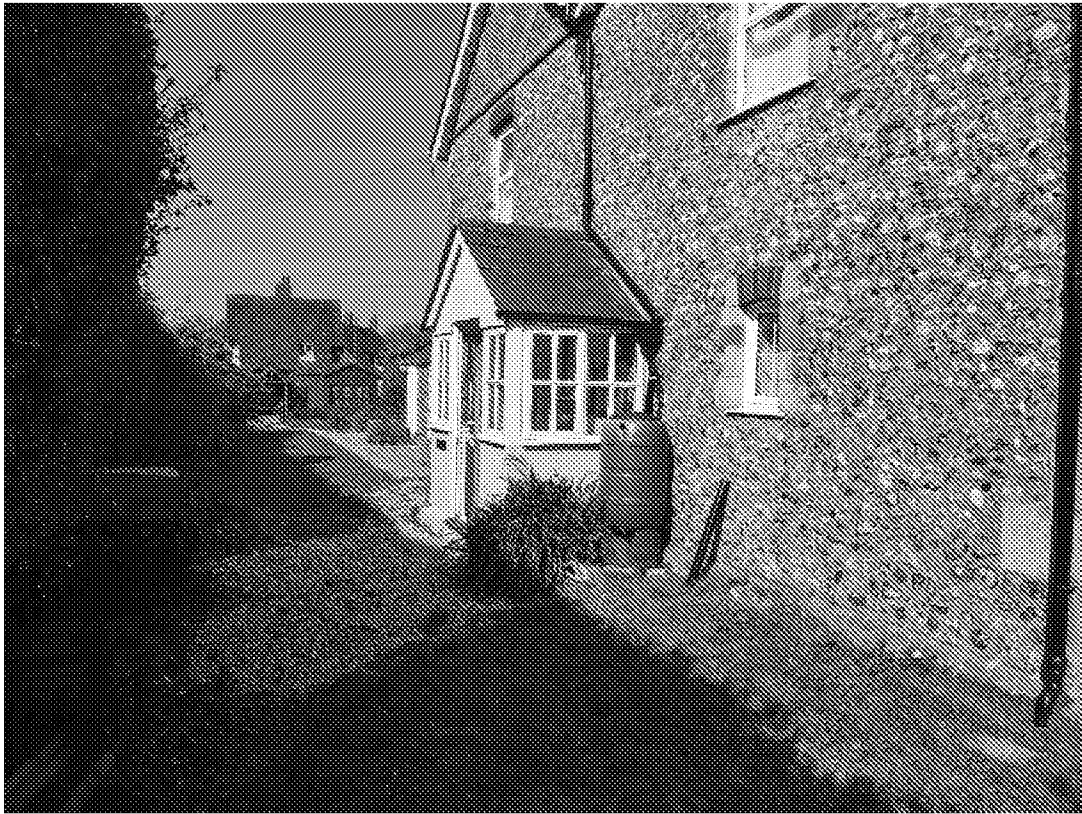
SIDE (SOUTH) ELEVATION, BOUNDARY HEDGE TO LEFT
