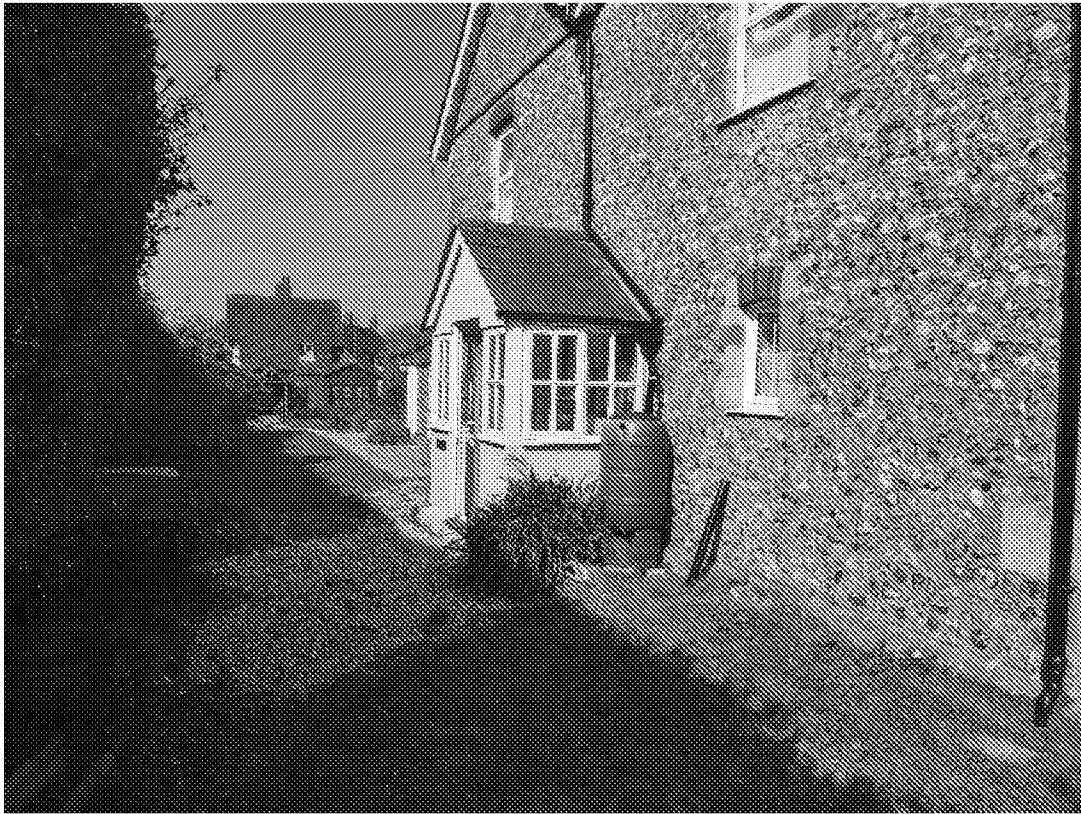
SIDE (SOUTH) ELEVATION, BOUNDARY HEDGE TO LEFT
