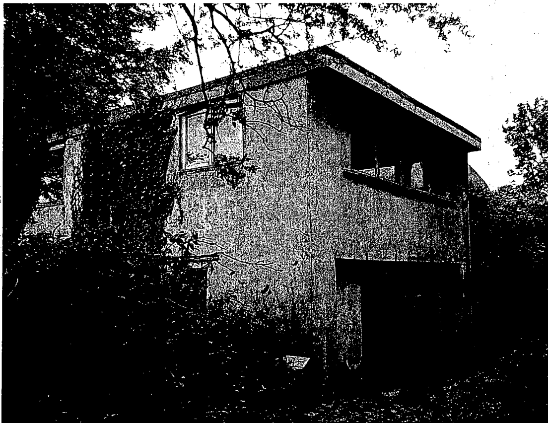
Photo 03 View of existing annex from Hoe Lane
