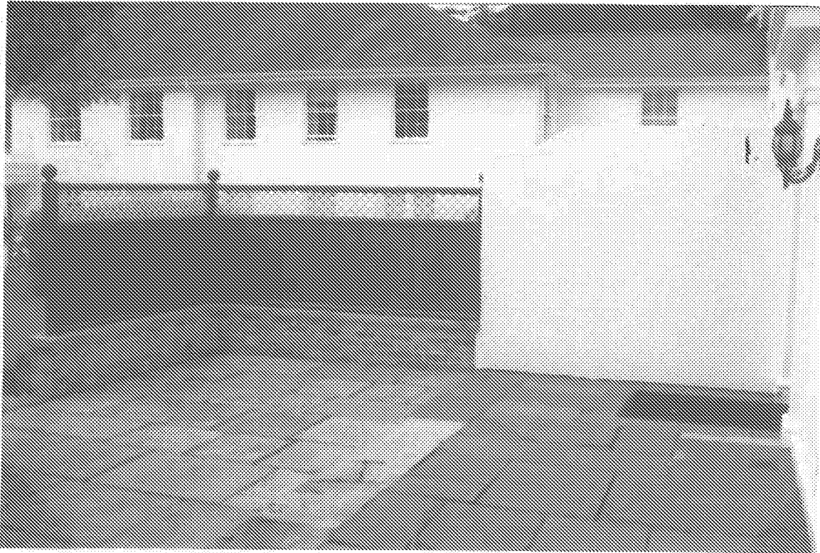
View of the Patio and replacement Privacy Screen. North West Corner, Facing North
