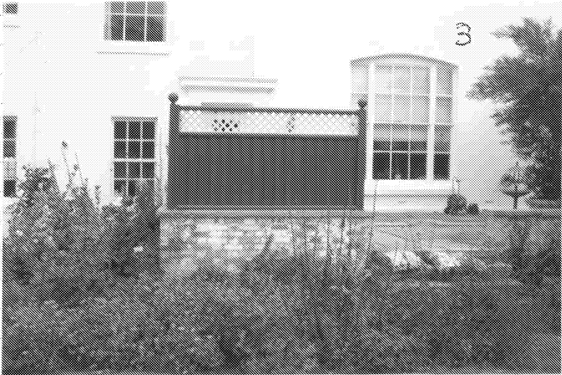
View of the Patio boundary Wall and Privacy Screen, North West side, facing East
