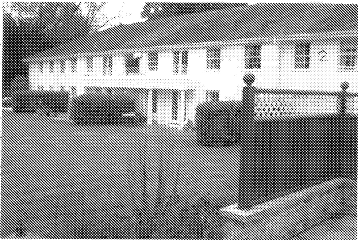
View of the low boundary Wall with replacement Privacy Screen affixed. West boundary of the patio, North end, facing North West
