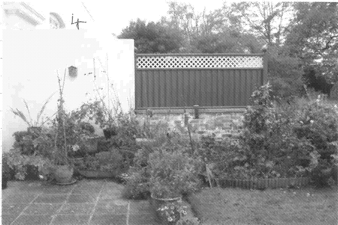
View of the North Patio boundary Wall and Privacy Screen, facing South.
