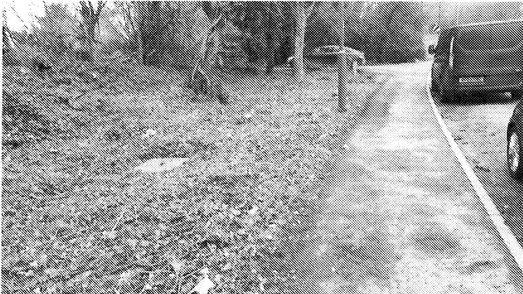
Existing footway on south side Arundel Road with existing vehicle site access in middle distance.
