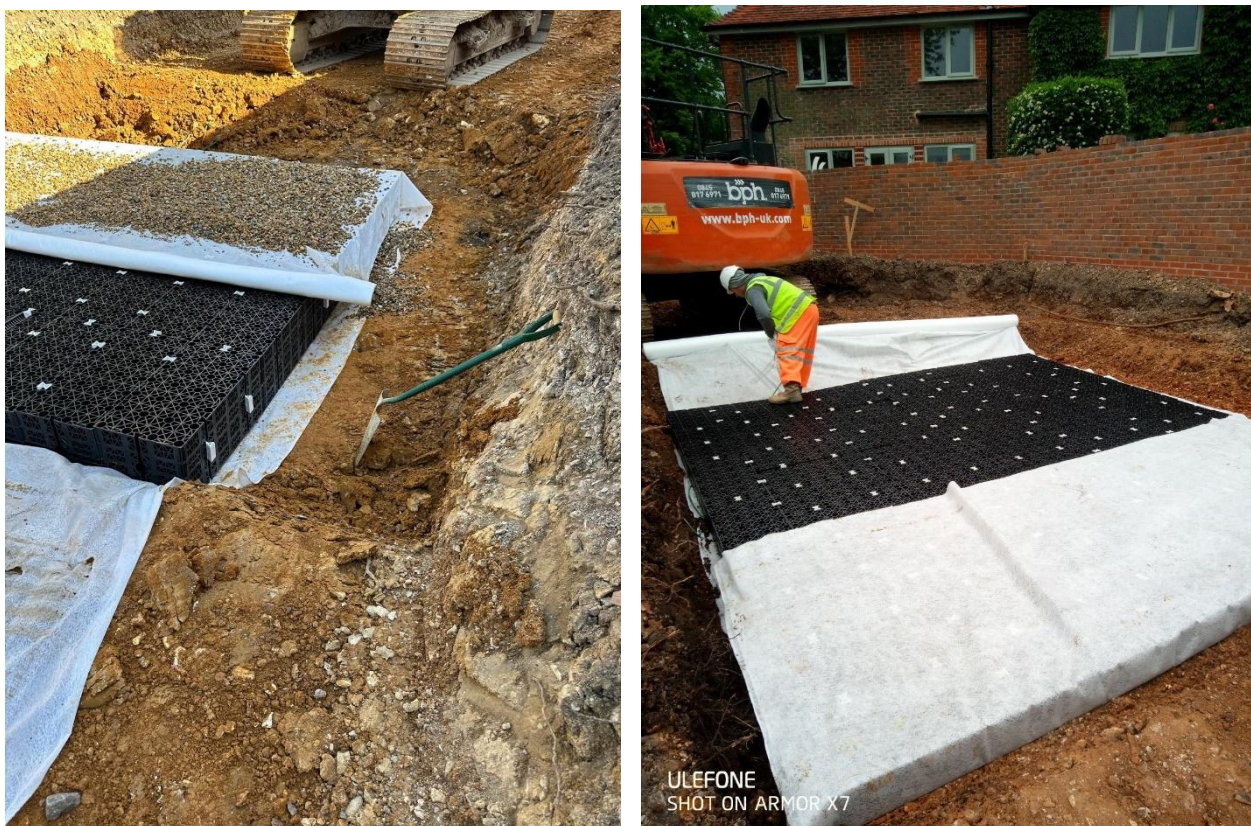
Fig 2. Installation of permavoids
