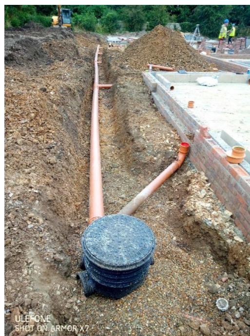
Fig 6. Surface water inspection chambers
