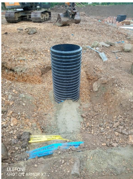
Fig 6. Surface water inspection chambers
