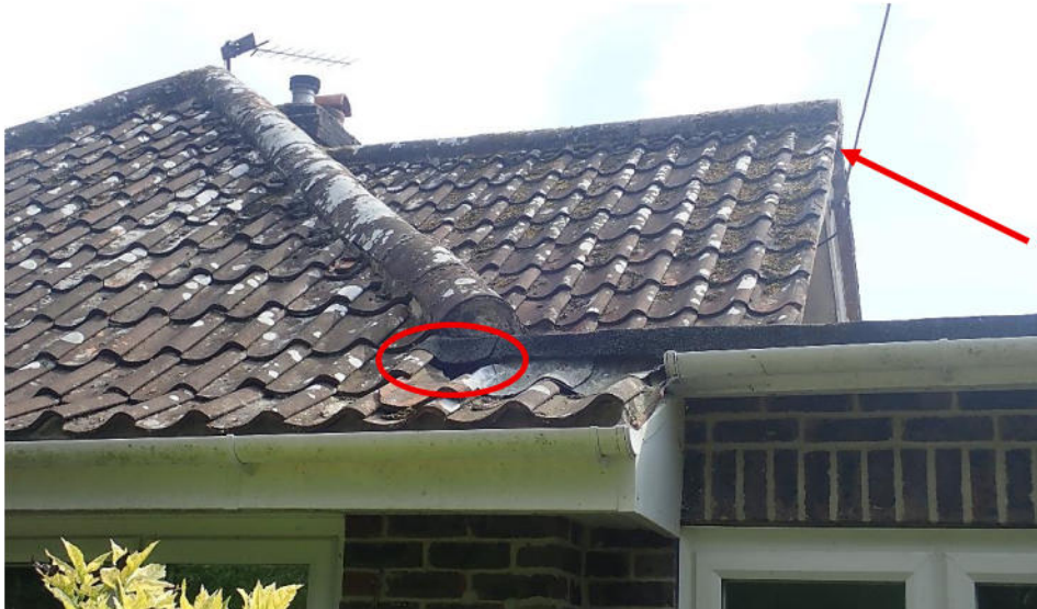
Fig. 5 – Front of property, gap where tile has slipped beneath flat-roofed section, circled Possible position of likely access point into area of roof void, where small numbers of bat droppings seen, arrowed (W) gable.
