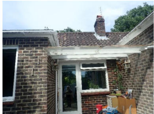
Fig. 5 – Front of property, gap where tile has slipped beneath flat-roofed section, circled Possible position of likely access point into area of roof void, where small numbers of bat droppings seen, arrowed (W) gable.
