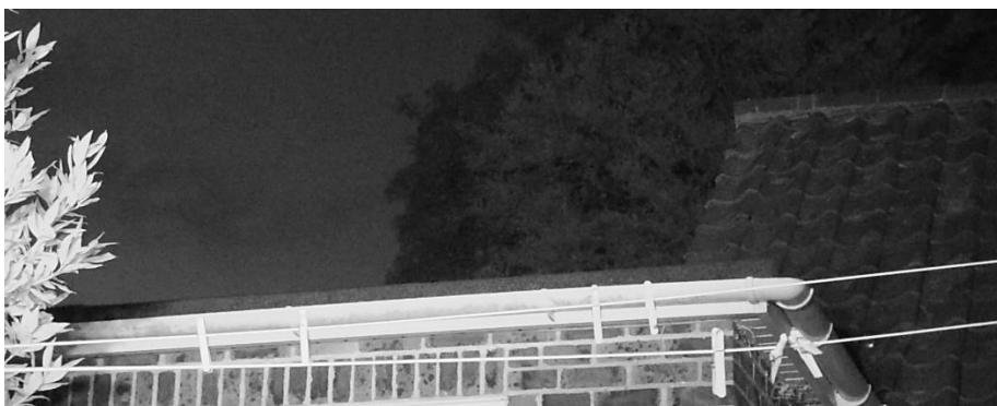
Fig. 16 – IR camera view from S (survey 1) – NW of house
