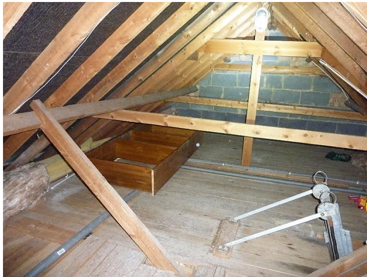
Fig. 9 – General view of roof void
