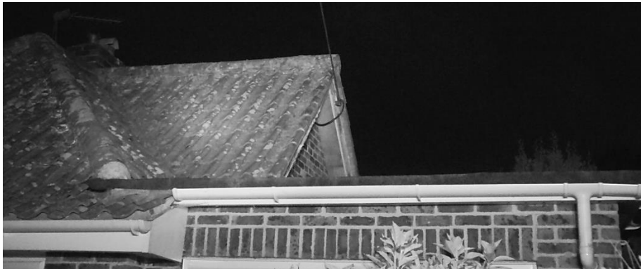
Fig. 15 – IR camera view from N (survey 1) – NW of house
