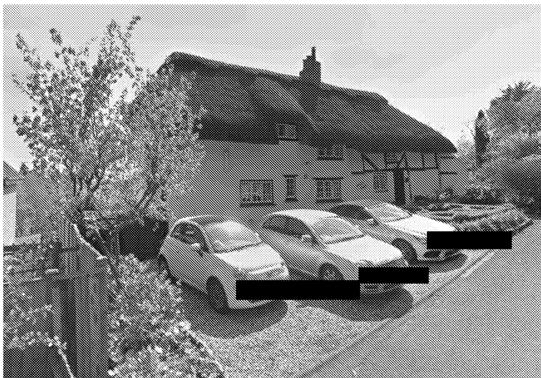
Plate 18. View south to Beam Ends
