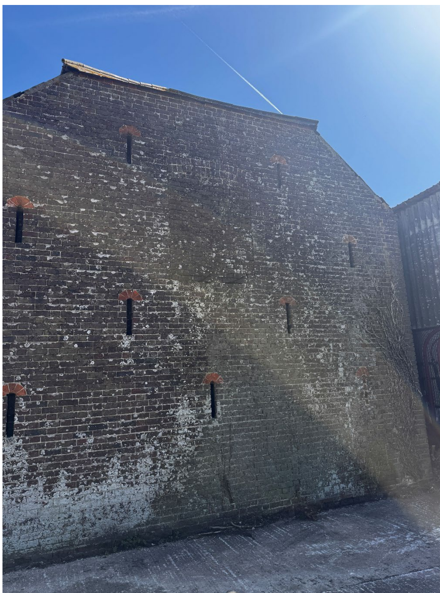
Figure 4 Gable Wall of Plot .
