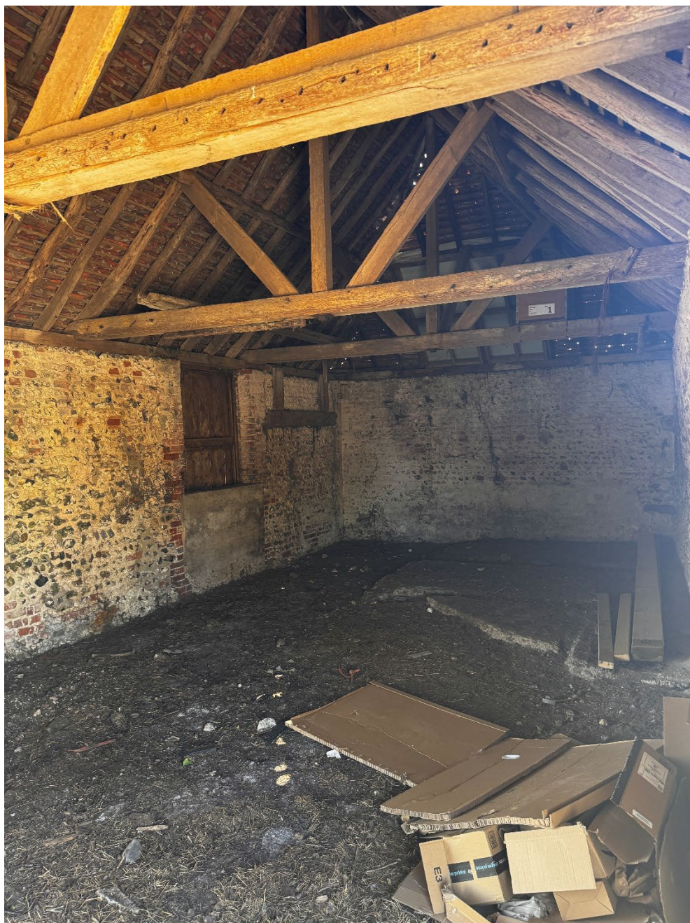
Figure 7 roof structure of plot 2
