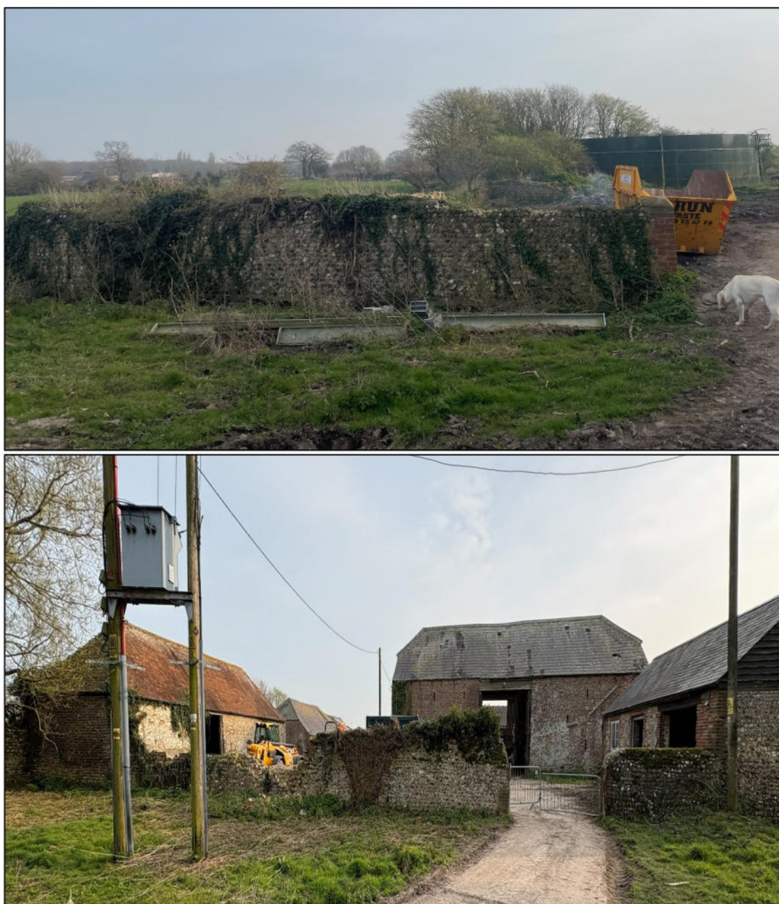
Figure 10: Existing flint walls will be retained and repaired with lime mortar
