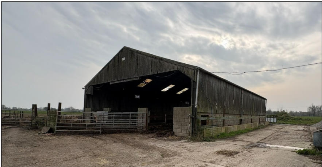
Figure 9: Plot 5 & 6, existing large modern barn to be demolished
