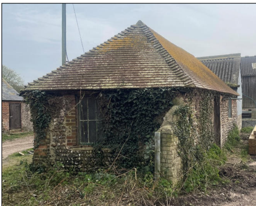
Figure 7: Vernacular outbuilding to be converted as ancillary office to serve dwelling in Plot 3
