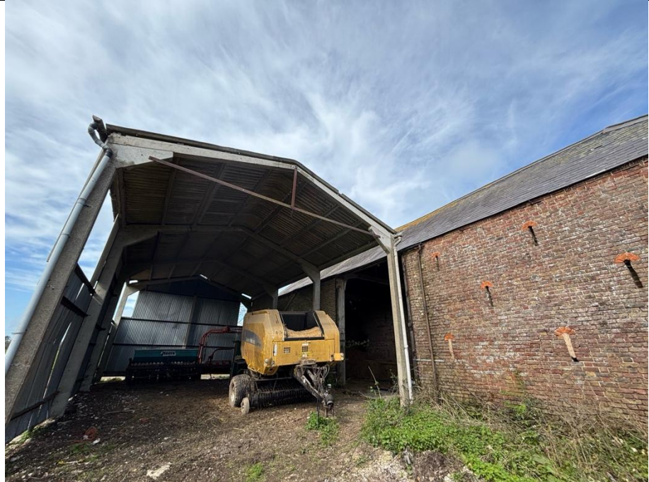
Photograph 14: Building B4 connected to the south of B3
