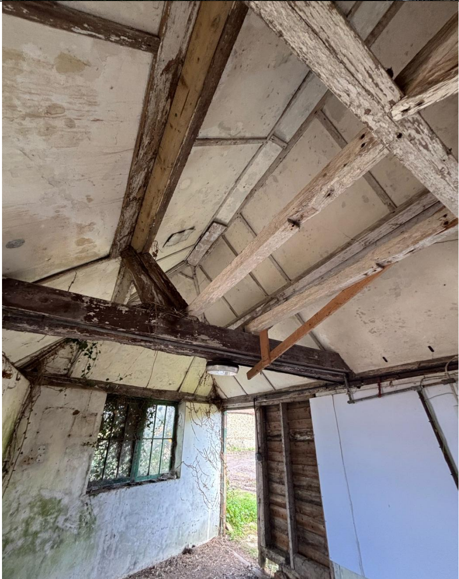
Photograph 16: Inside building B5
