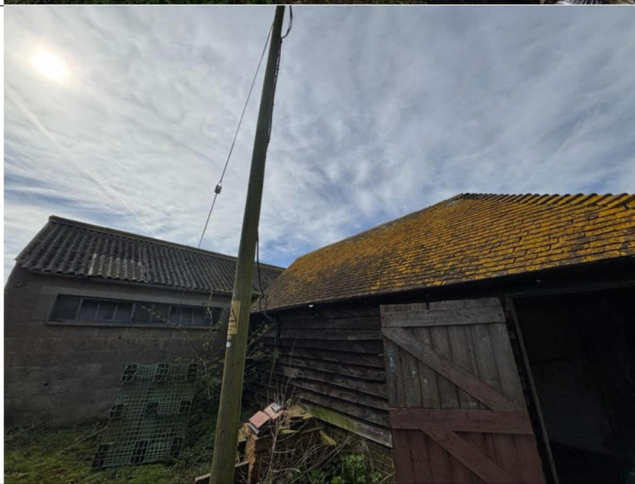
Photograph 6: Wooden cladding on side of B5 and B6 breeze block structure and corrugated metal roof
