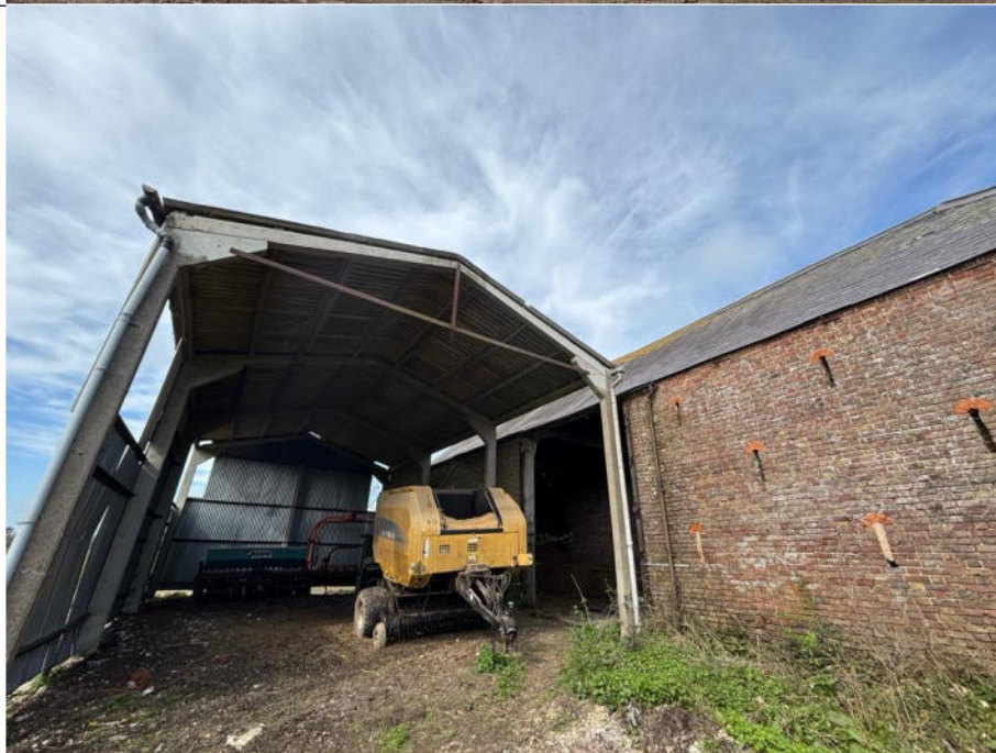
Photograph 4: Building B4 connected to the south of B3
