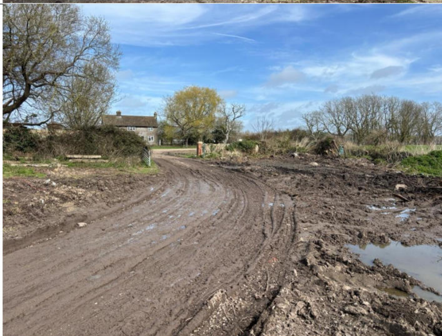
Photograph 12: Artificial unvegetated unsealed surface under regular disturbance
