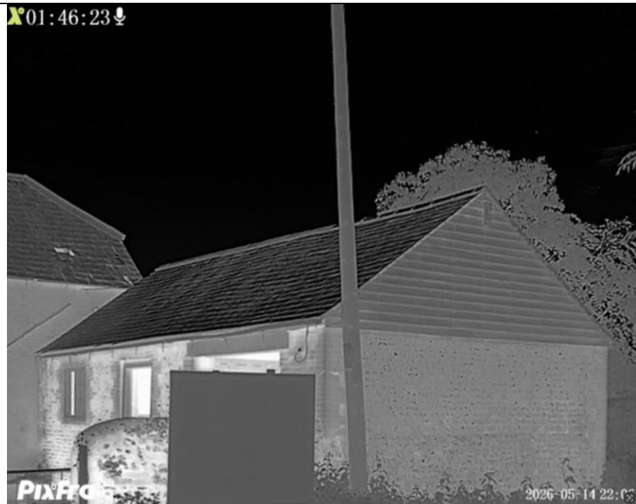
Figure 7: Screenshot of Thermal footage to the north-east of B2 on 14/05/26
