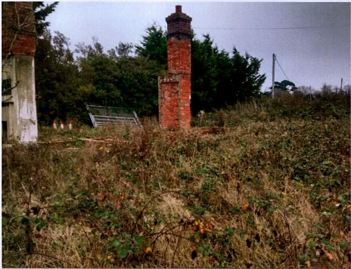
Photo 3: Former bungalow site with bramble re-growth and cypress-hedge at entrance
