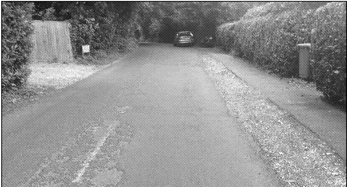
View looking west along Wandleys Lane
