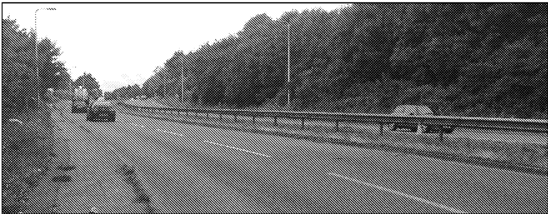
View looking west from the A29 roundabout on the A27
