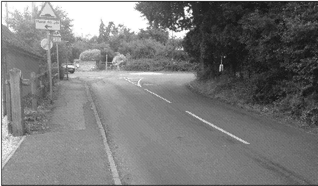
View looking north along West Walberton Lane towards Arundel Road
