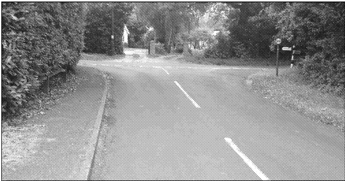
View looking along Wandleys Lane towards junction with West Walberton Lane
