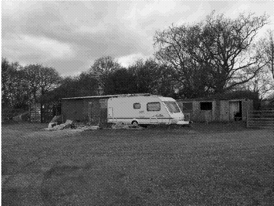
Figure 17: The group of non-descript and derelict buildings located near the Site's entrance gate.
