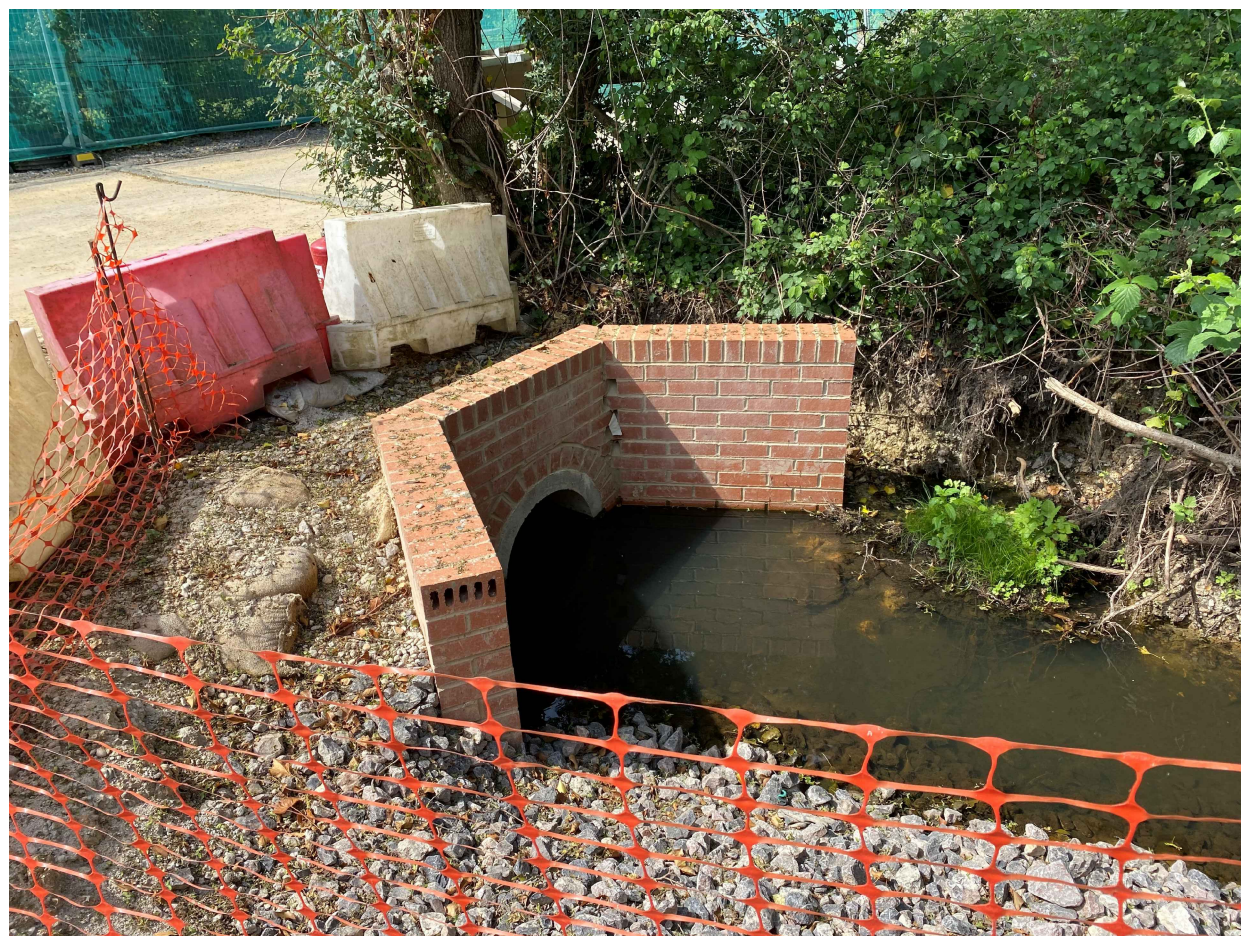
SIMPLE HEADWALL ELEVATION (INLET) As built site photo for information
