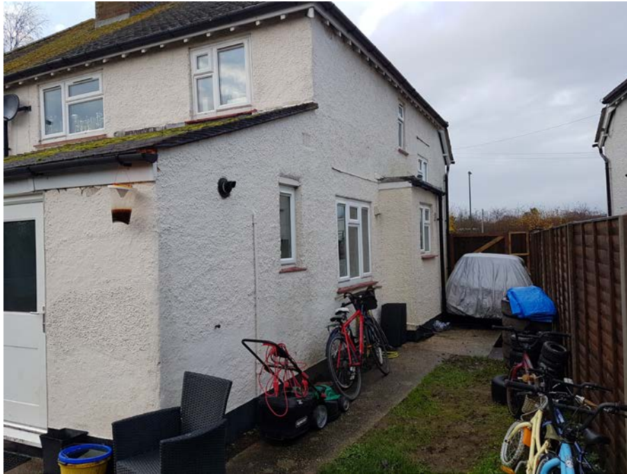
3: View of side of property from SE corner
