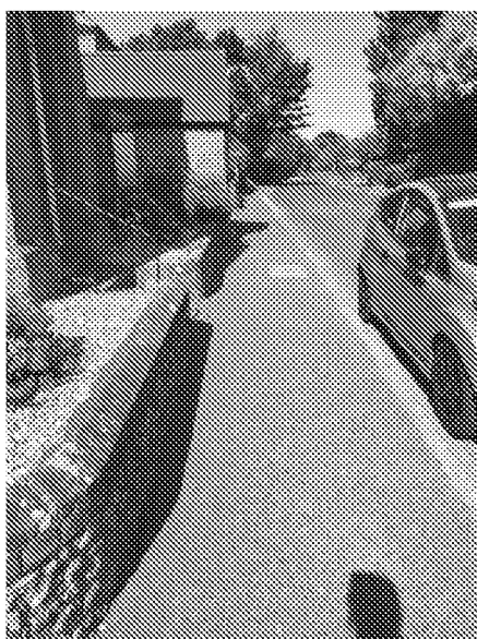
Photograph 11: Southern Footway On The Street
