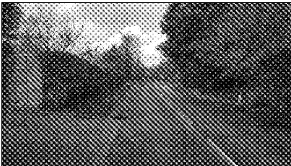
Plate 8: View N towards Site from conservation area boundary in Tye Lane
