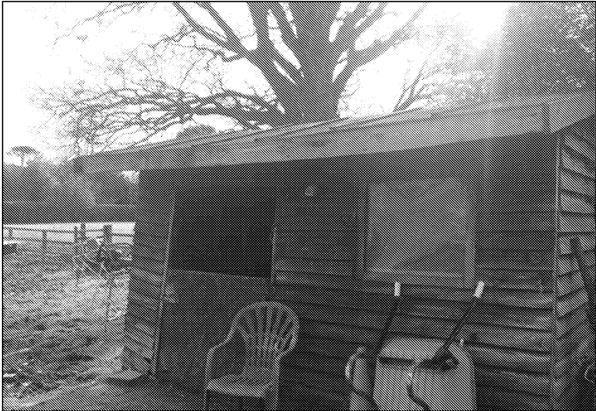
Figure 15. Building 3 within the site used for stabling horses.
