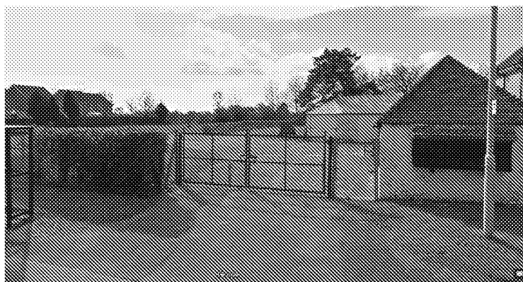
Figure 1 - Photograph of the existing access off Arundel Road
