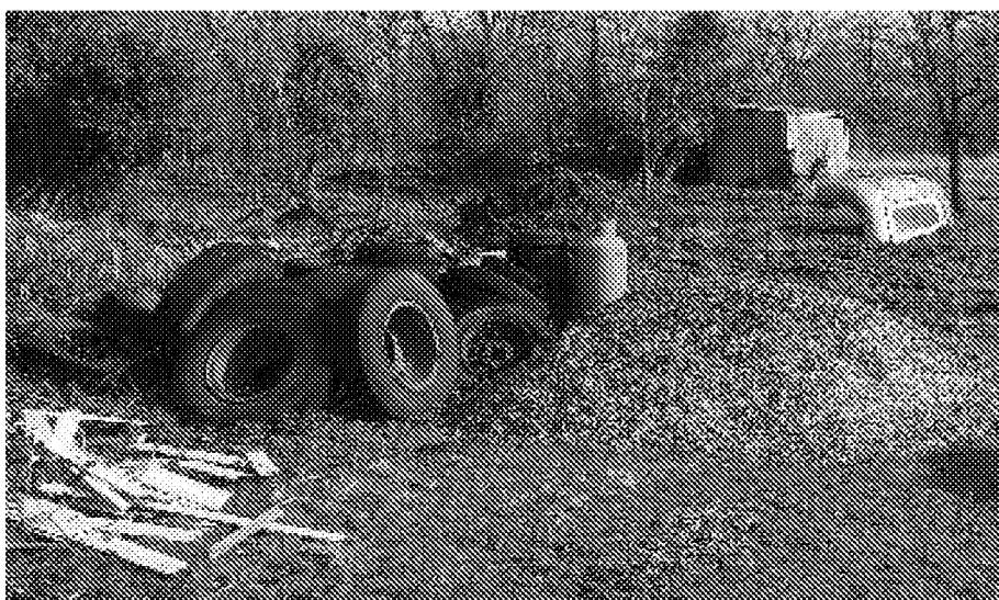
Figure 4: Piles of refuse and woodchippings neat the site entrance.
