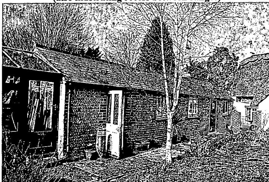
EAST ELEVATION OF ANNEXE
