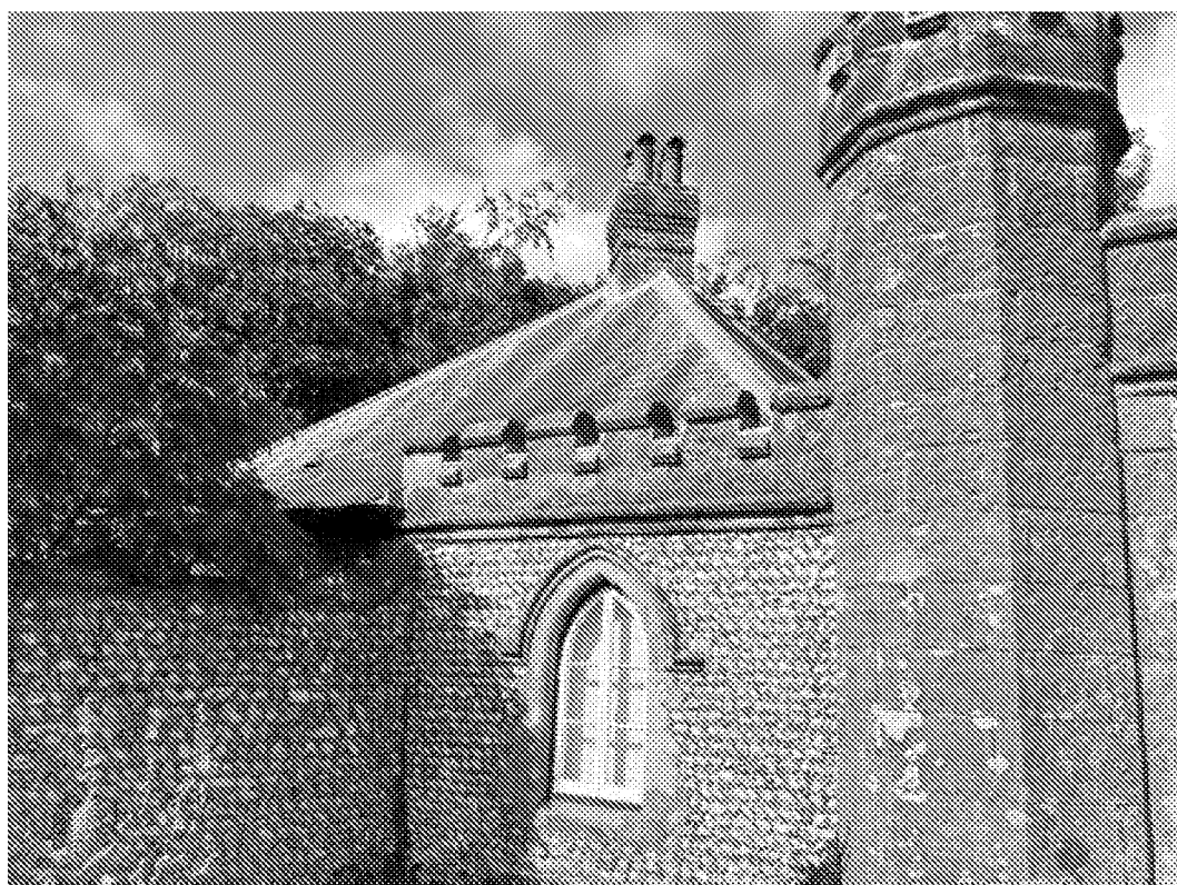
Figure 13: View of Lodge roof over the Gateway wall
