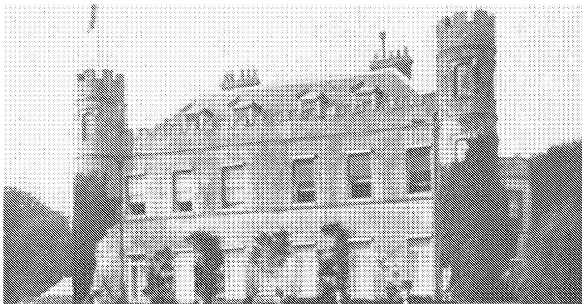
Figure 10: Slindon house c.1918
