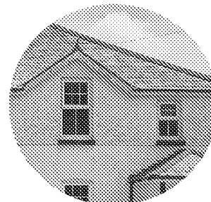
Gablet and smaller window below dropped eaves
