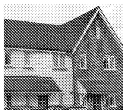
Variety of roof forms, including gables and hipped roofs
