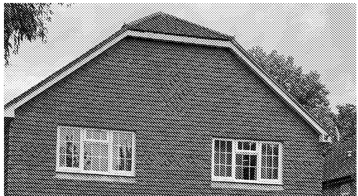
Barn hipped roofs
