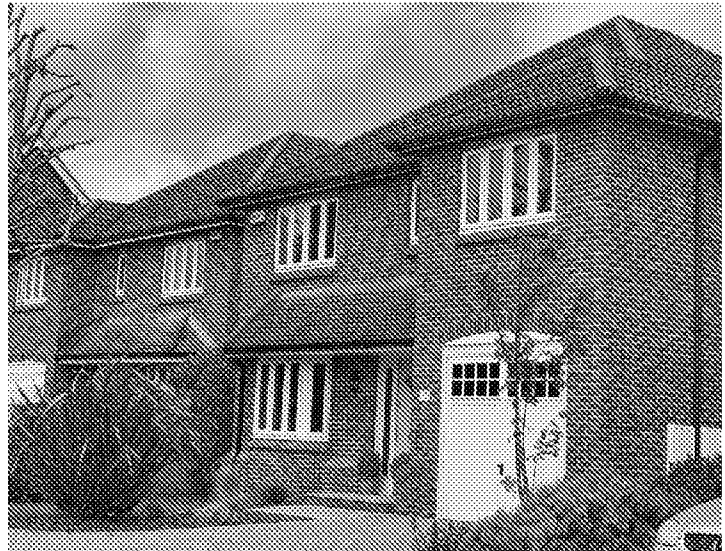
Hipped roof properties
