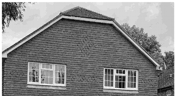
Barn hipped roofs
