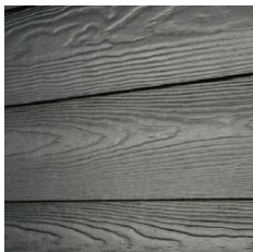
Black weatherboard cladding
