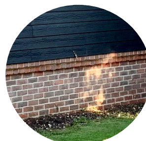
Low level contrasting brick band
