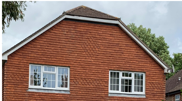
Barn hipped roofs
