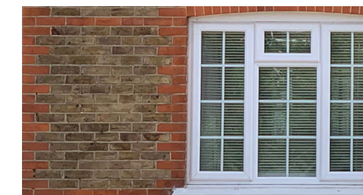
Buff brick with red quoins and side hung windows
