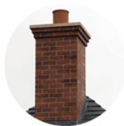
Brick clad chimney (cottages and flint properties only)
