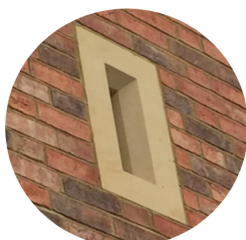
Stone gable vent
