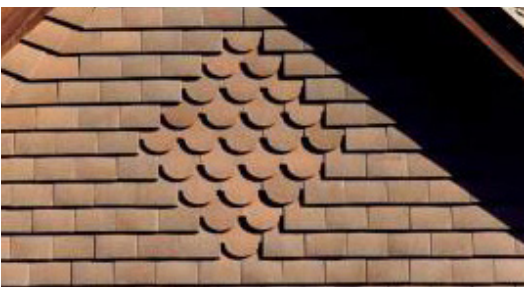
Decorative hanging tiles as features
