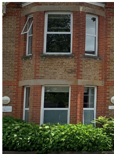
Claremont Gardens: Splayed bay windows featuring red brick quoins, stone cills and heads
