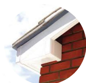
Boxed eave with white barge board
