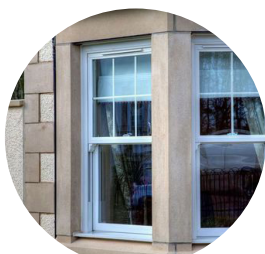
Sliding sash style window
