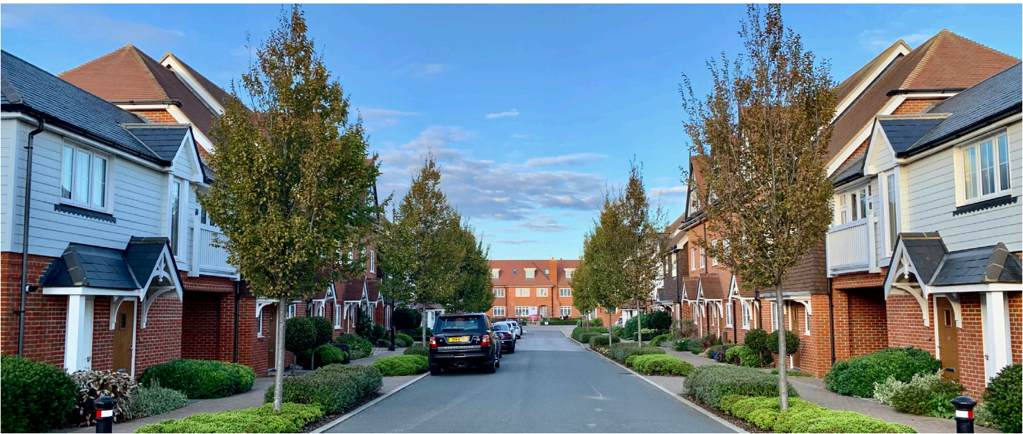
Bersted Park: A landscaped street leading into sequenced tree planting. A variation in building height, roof forms and facade treatment adds interest to the street scene.
