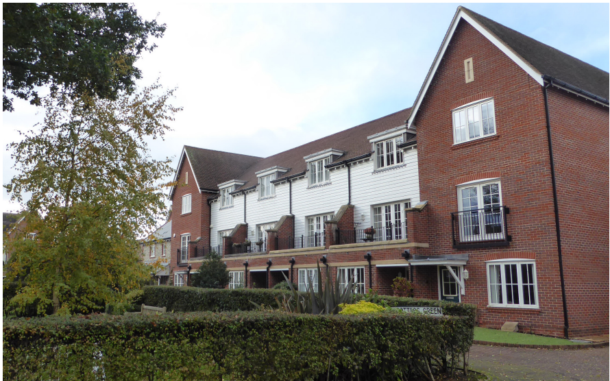
Westhampnett: Prominent gable frontages addressing tree lined street with small landscaped frontages
