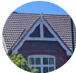
King truss with decorative barge board
