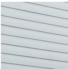
Pale weatherboard cladding
