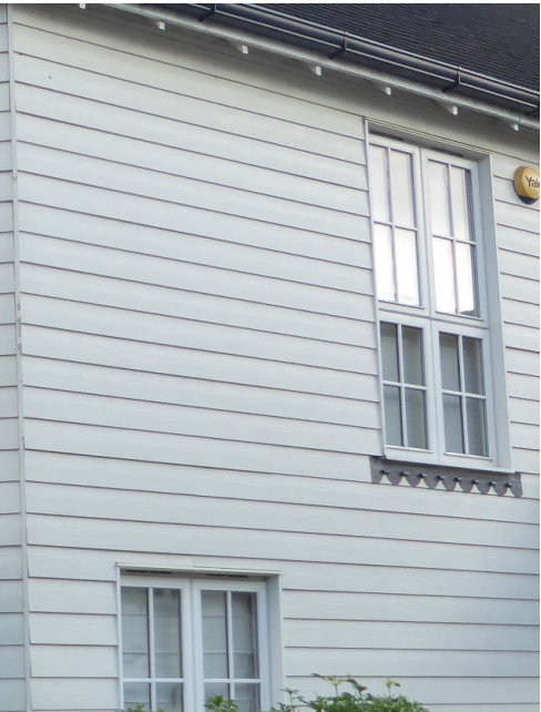
Pale weatherboard cladding
