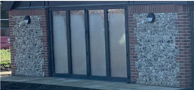
Full height glass windows on flint with brick quoins
