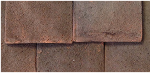
Plain style roof tiles and vertical hanging tiles
