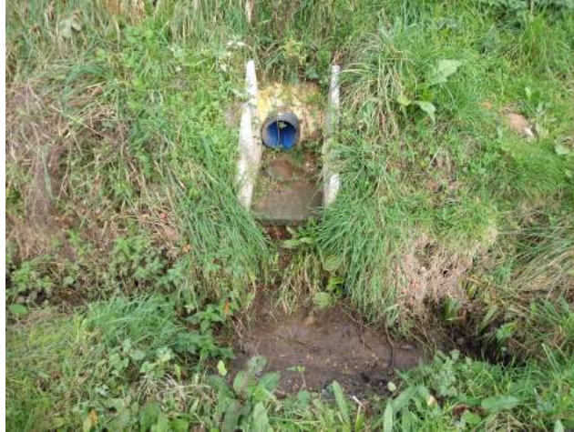
Outfall to ditch
