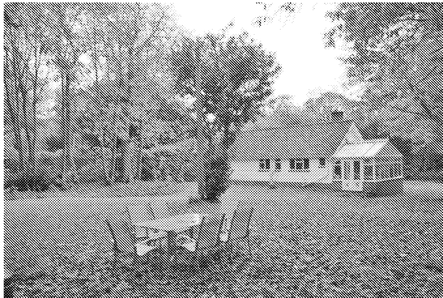
The rear of the existing cottage
