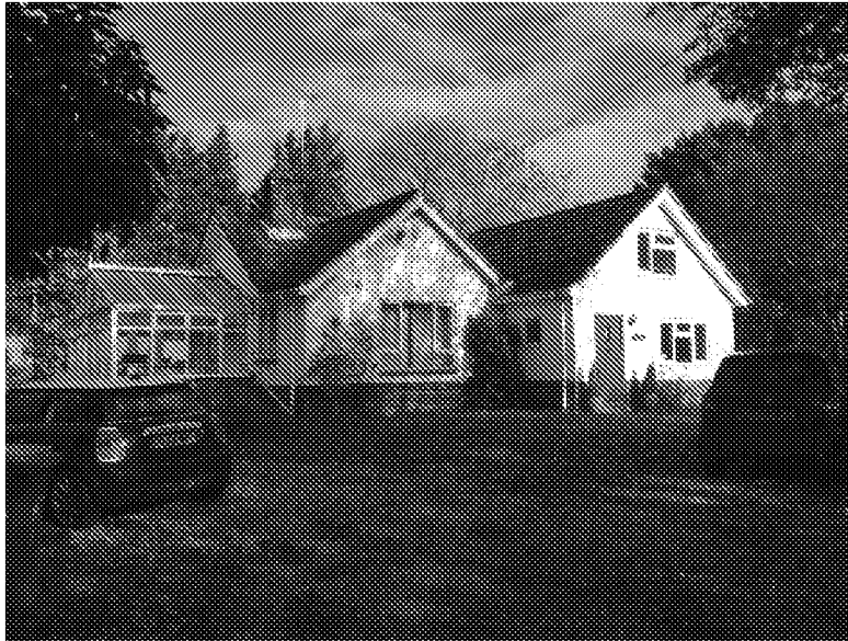
The existing front elevation
