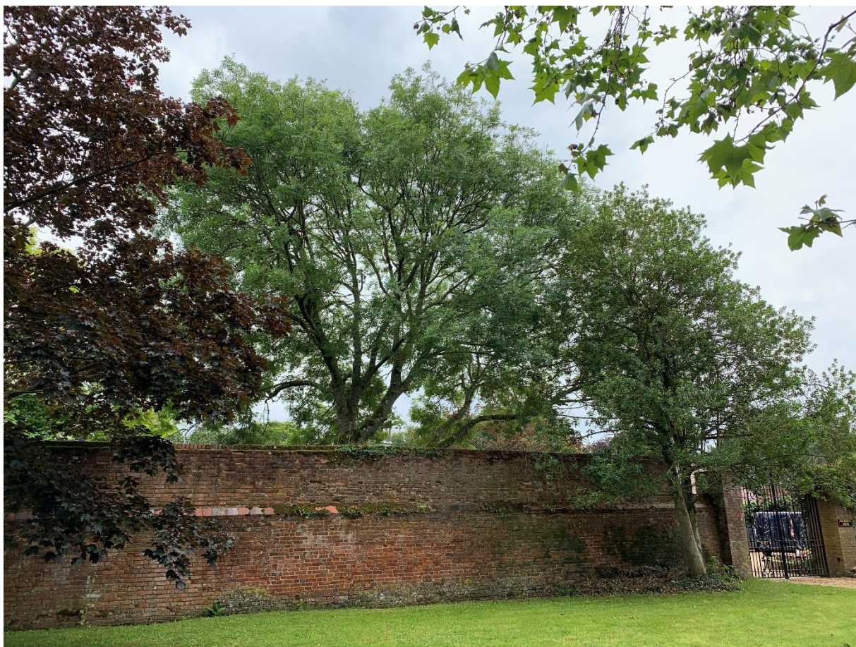
Fig.1. – T1 ash behind boundary wall, from driveway to Walberton House.
