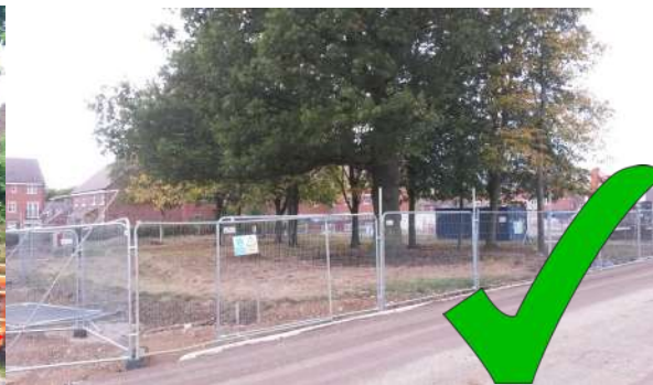
Tree Protection Fencing which has been erected prior to the commencement of any site works and the correct signage has been provided to clearly highlight that this is a protected zone.
