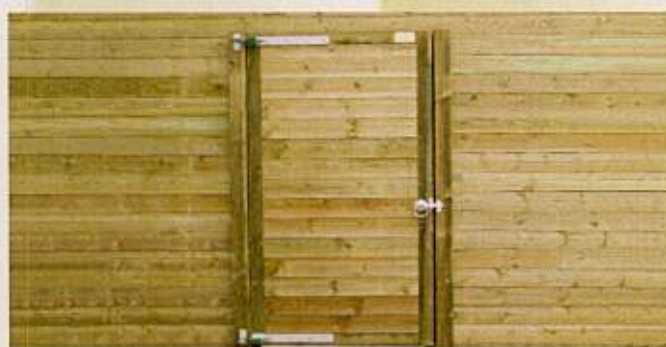
2m high x 1m wide gate within 3m high Jakoustic fencing
