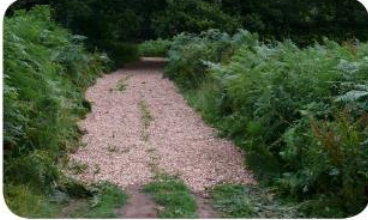
Step 1: Prepare Surface
