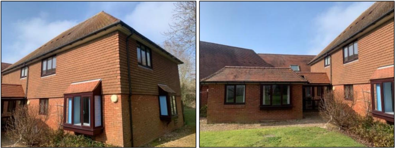
Photograph 15a & b. View's of the north-eastern extension of Russett Cottage's and the pitched entranceway connecting this to the main building.
