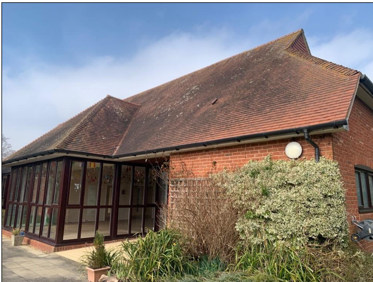
Photograph 13. Southern elevation of Hive and Apple Juice Building, viewed from the south-east corner.
