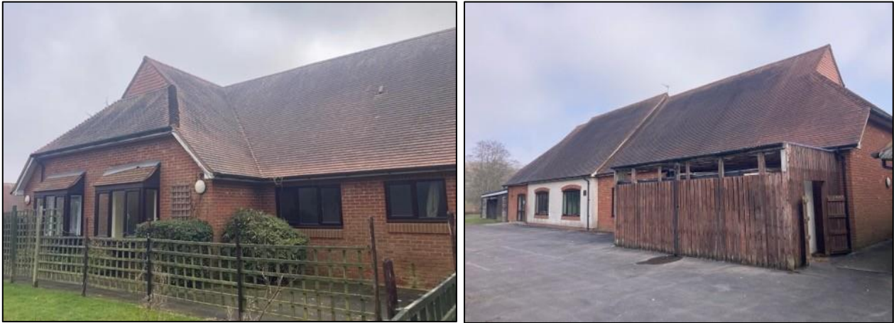
Photograph 18a & 18b. View of the eastern and western elevations of Day Centre.
