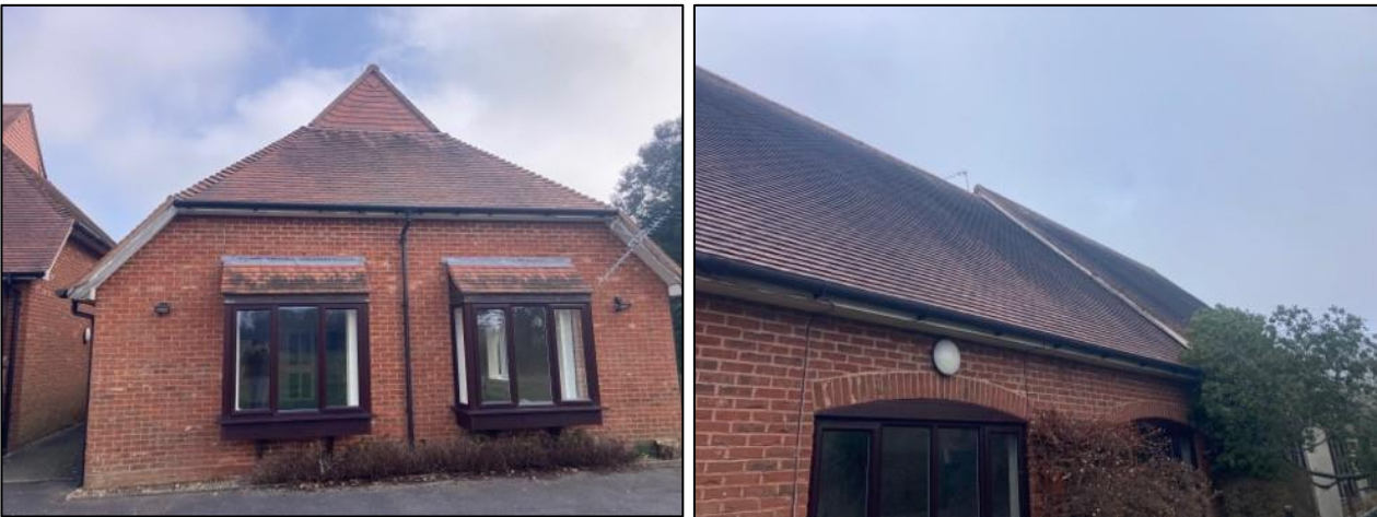
Photograph 19a & 19b. View of the western elevation of Day Centre and example of the roof of Day Centre, showing limited suitability for bats.
