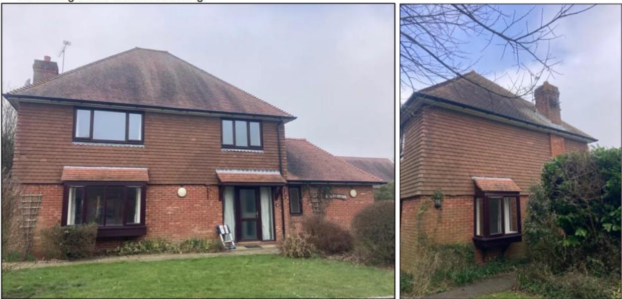
Photograph 16a & 16b. The eastern and southern elevations of Bramley Cottage.
