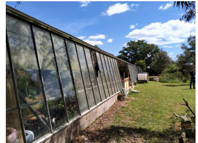
FIGURE 6: SOUTH FACE OF FRAMPTON FERGUSON GLASSHOUSE
