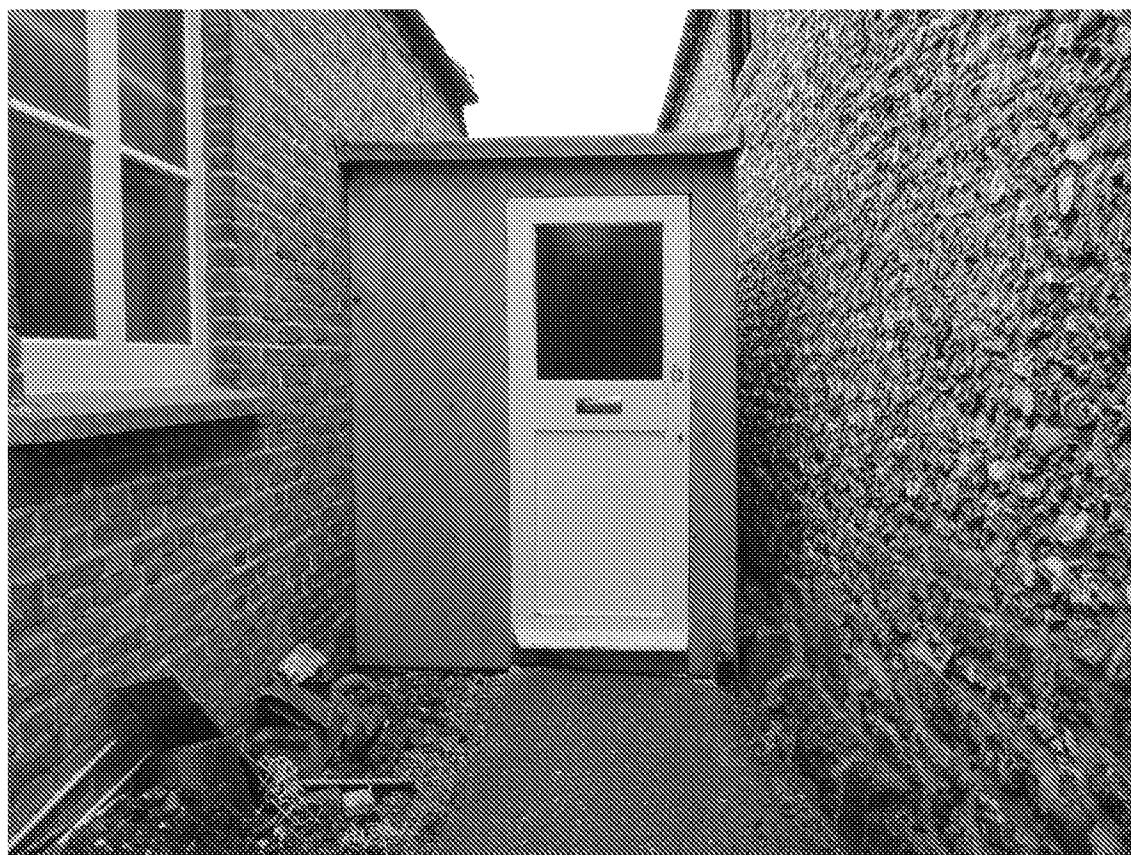
Picture – temporary structure in place.
