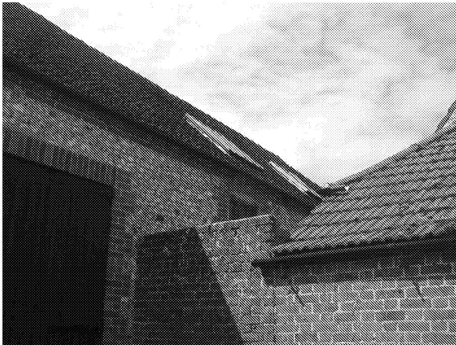
Picture – The view to the rear of the building showing the wall that will visually shield the new extension.
