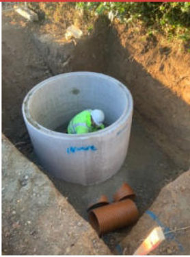
S2 MH BEING BENCHED
