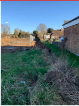
DITCH EXCAVATION BY FIELD CLOSE FOR CATCH PIT 70.
