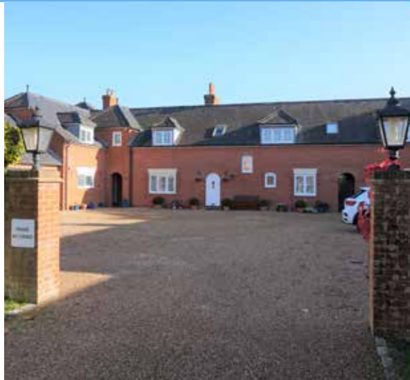
Oving: A series of terrace cottages framing shared courtyard space
