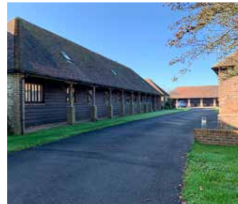
Tangmere: Access driveway to courtyard enclosed by open side elevation to barn
