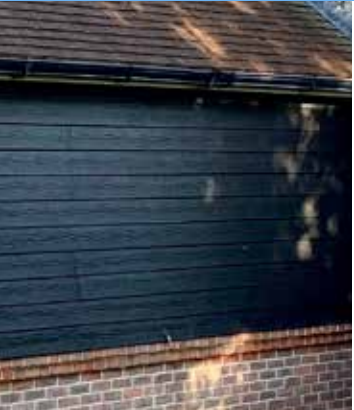
Black weatherboard cladding with brick plinth
