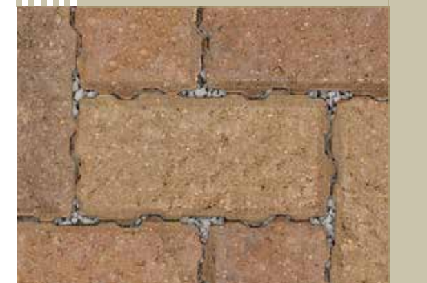
Carriageway surface materials references
