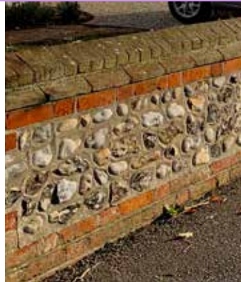
Low rise flint and brick headed boundary wall
