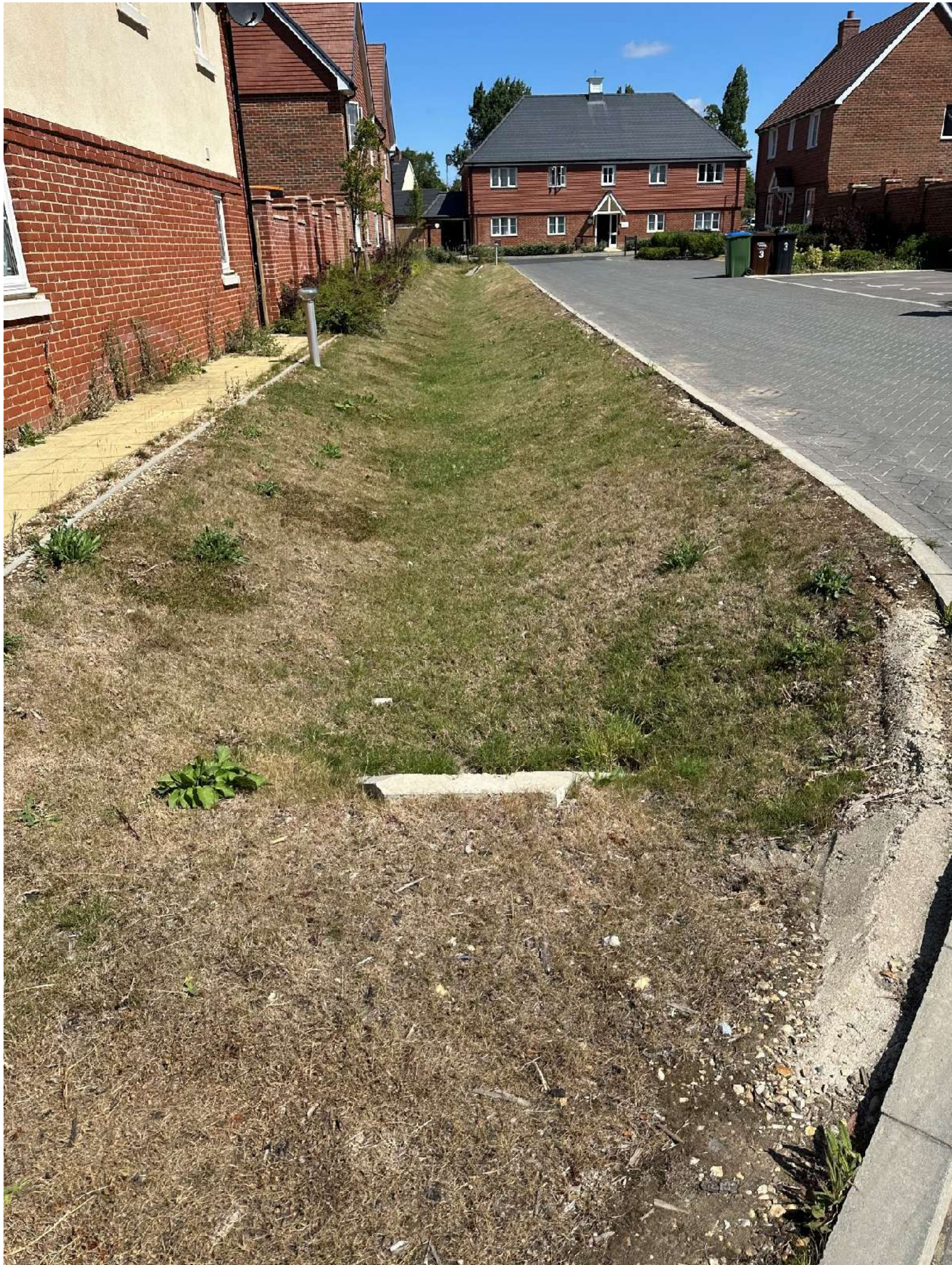
Swale X – 16 th July 2025 - complete and functioning
