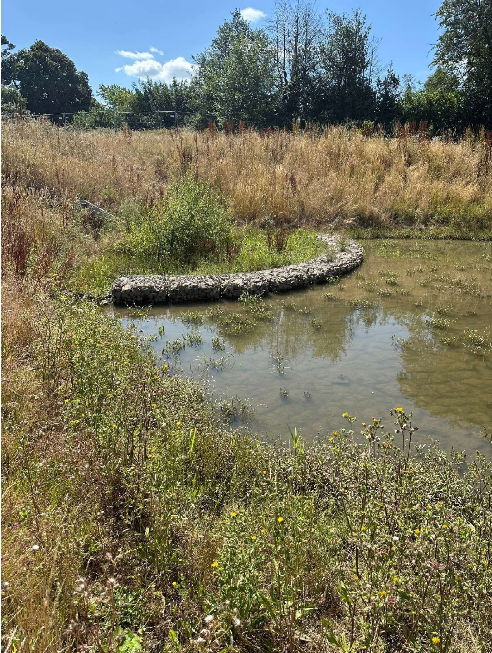
Western Basin – 16 th July 2025 - complete and functioning
