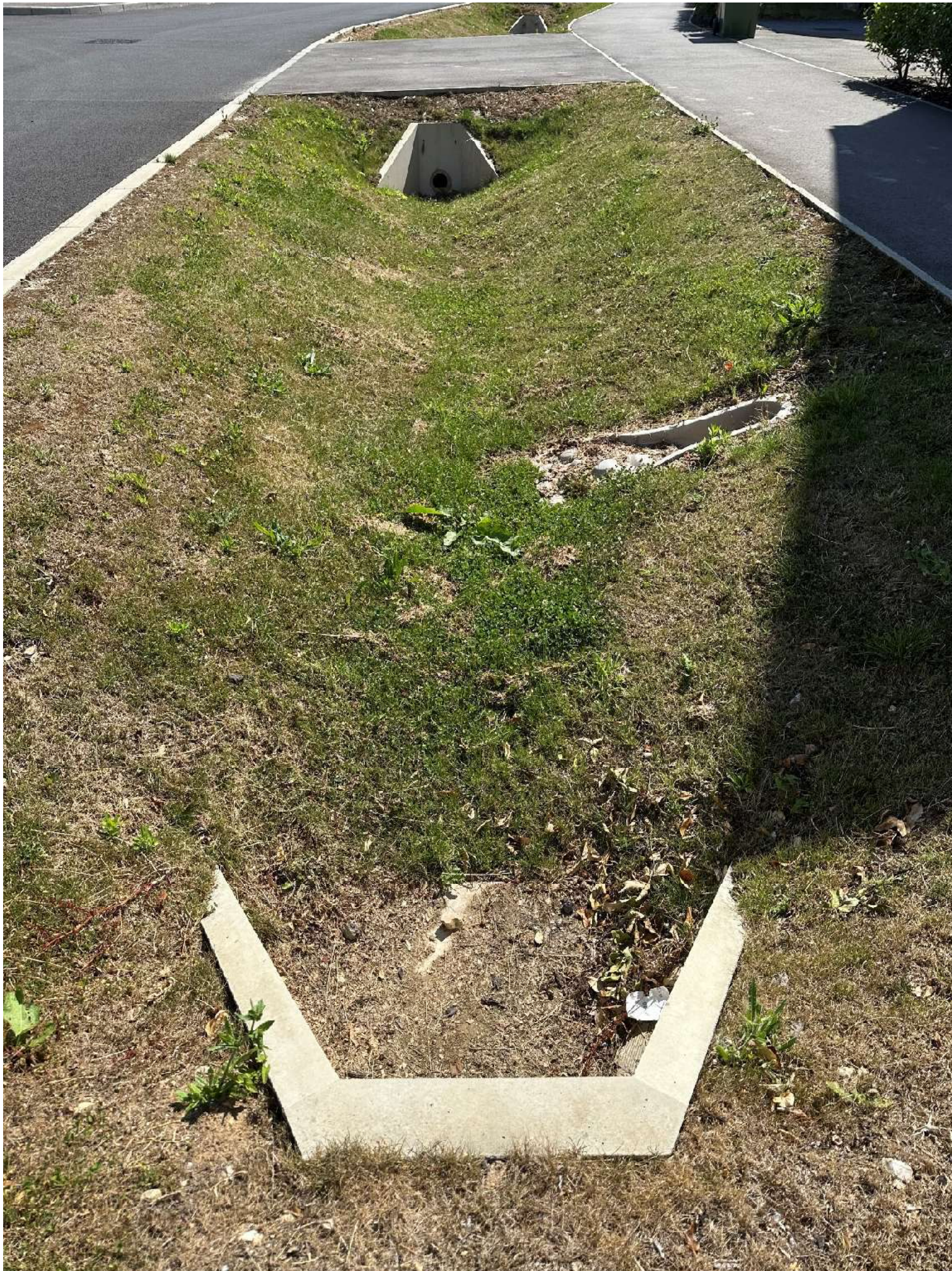
Swale W – 16 th July 2025 - complete and functioning
