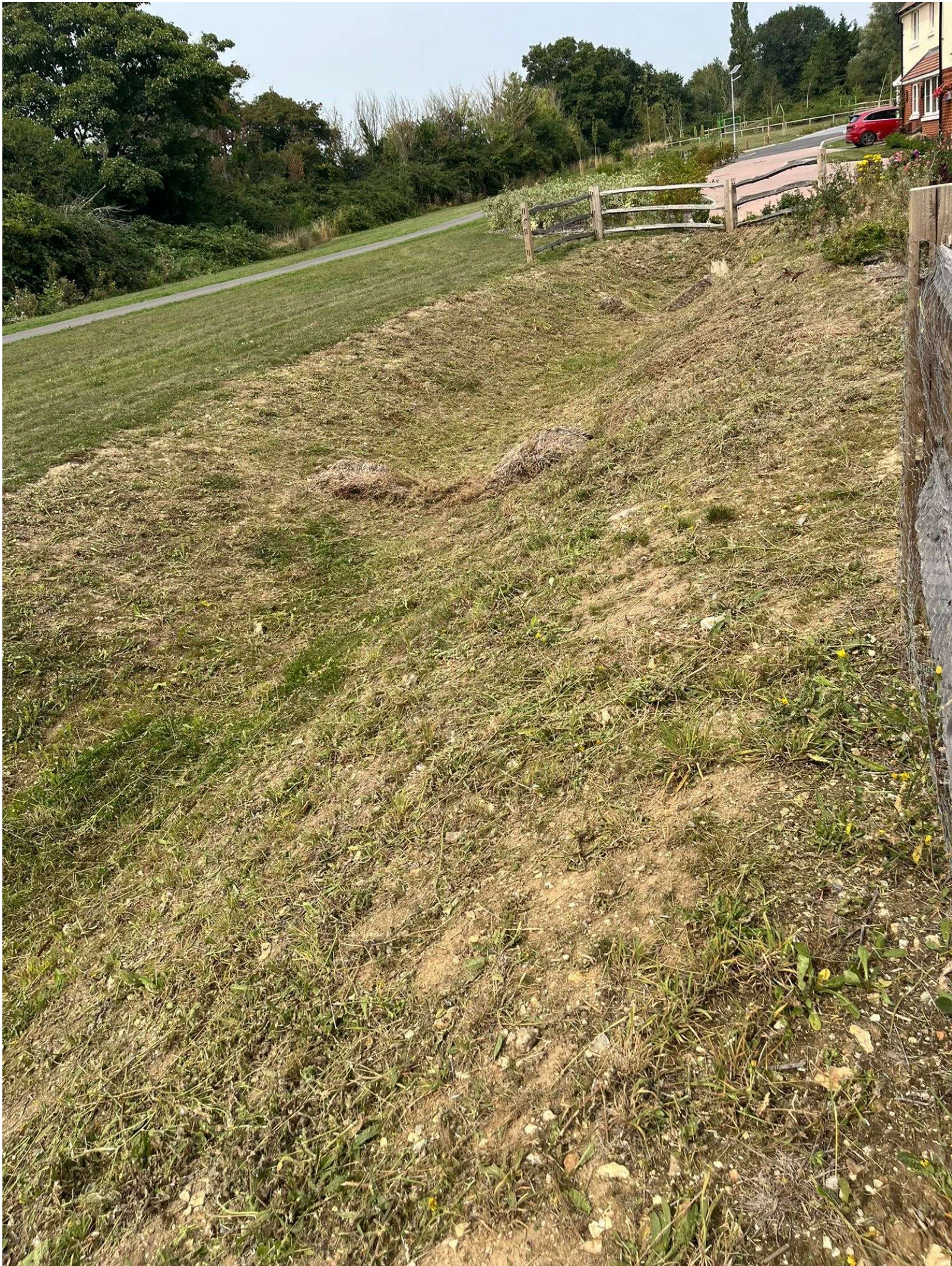
Swale A/B – 16 th July 2025 - complete and functioning
