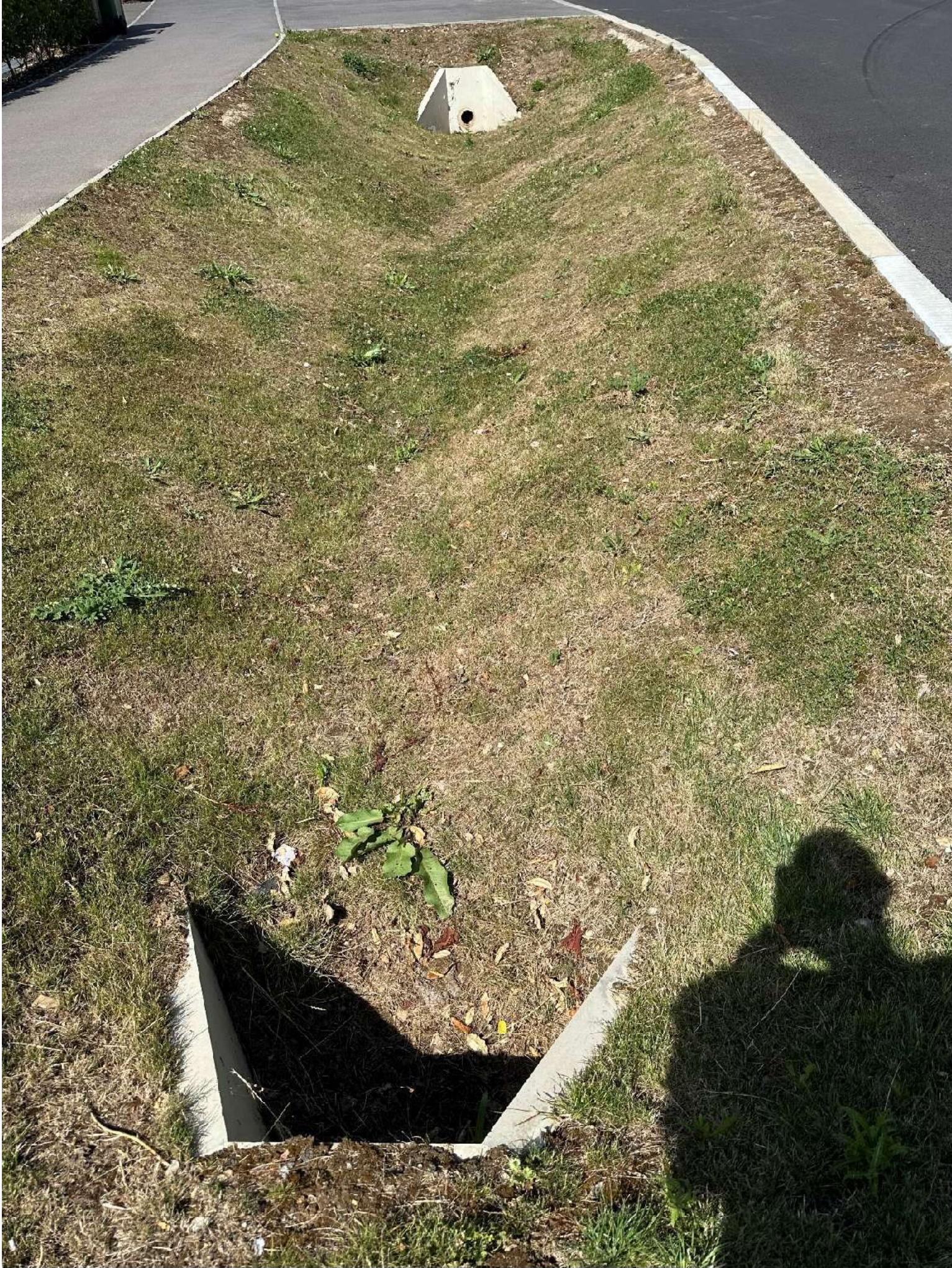
Swale V – 16 th July 2025 - complete and functioning
