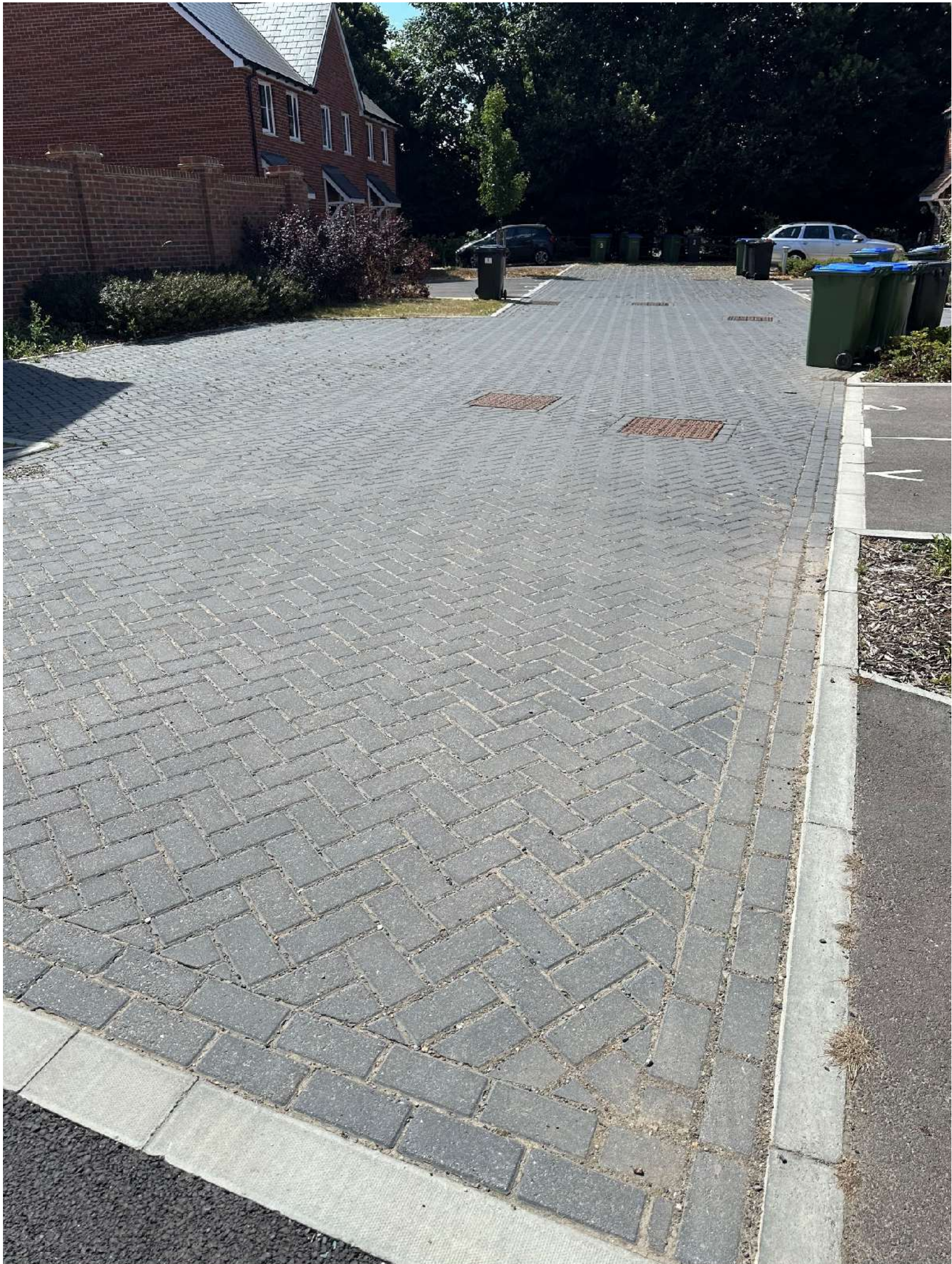
Private parking and Stedman Avenue – 16 th July 2025 - complete and functioning
