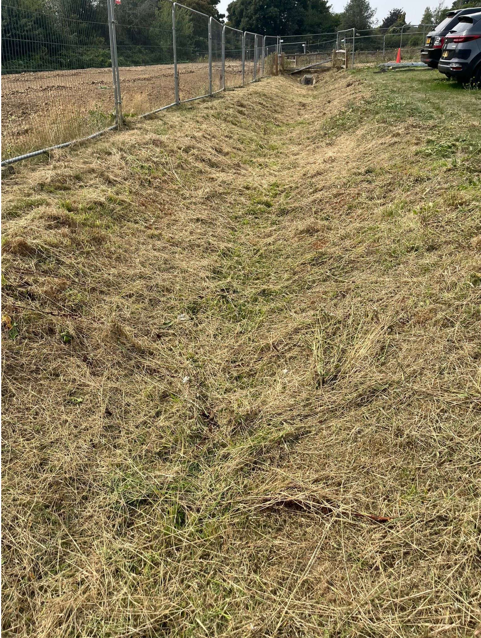
Swale Z – 16 th July 2025 - complete and functioning
