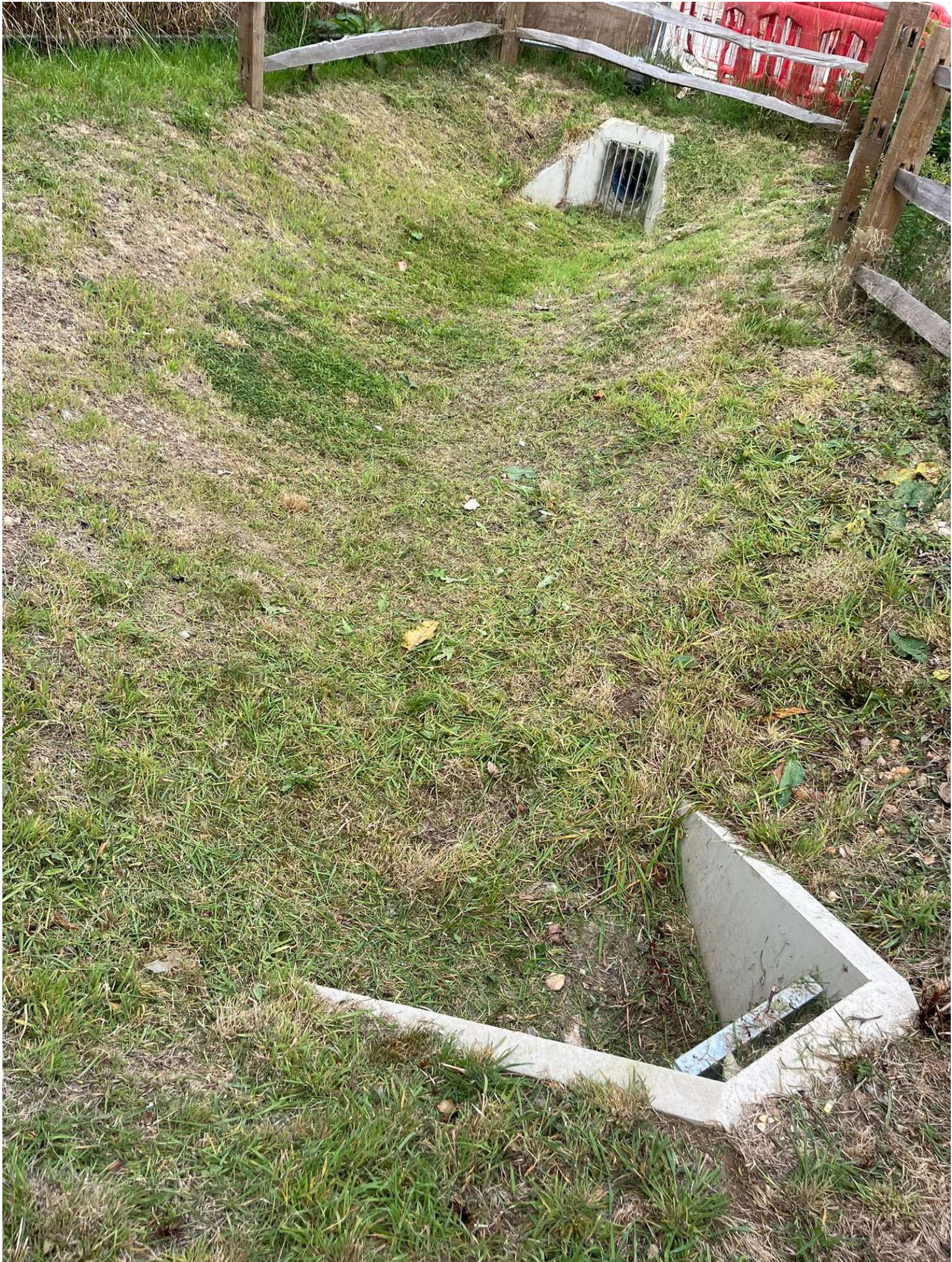
Swale Y – 16 th July 2025 - complete and functioning
