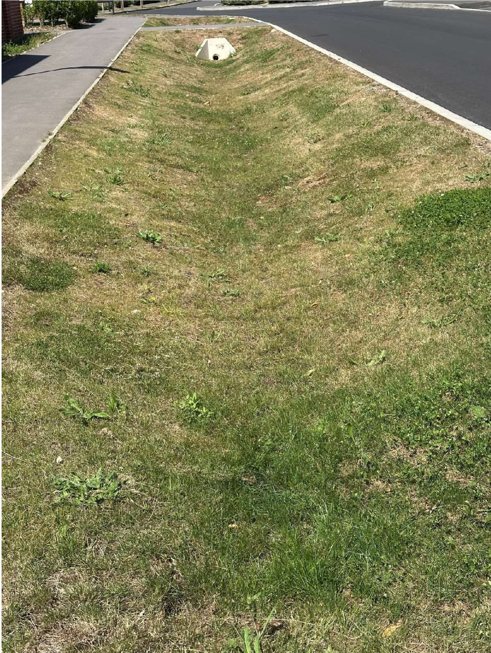
Swale U – 16 th July 2025 - complete and functioning
