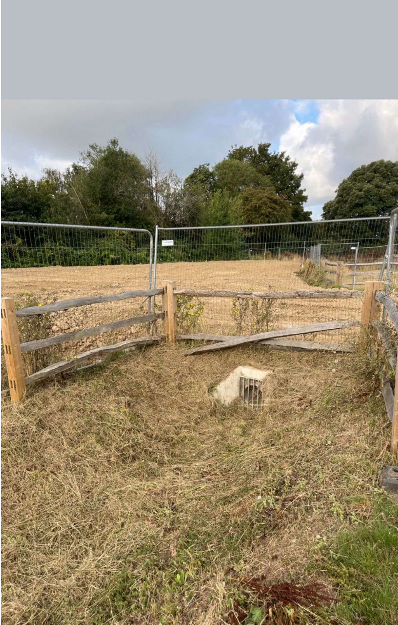
Headwall 3C – 16 th July 2025 - complete and functioning
