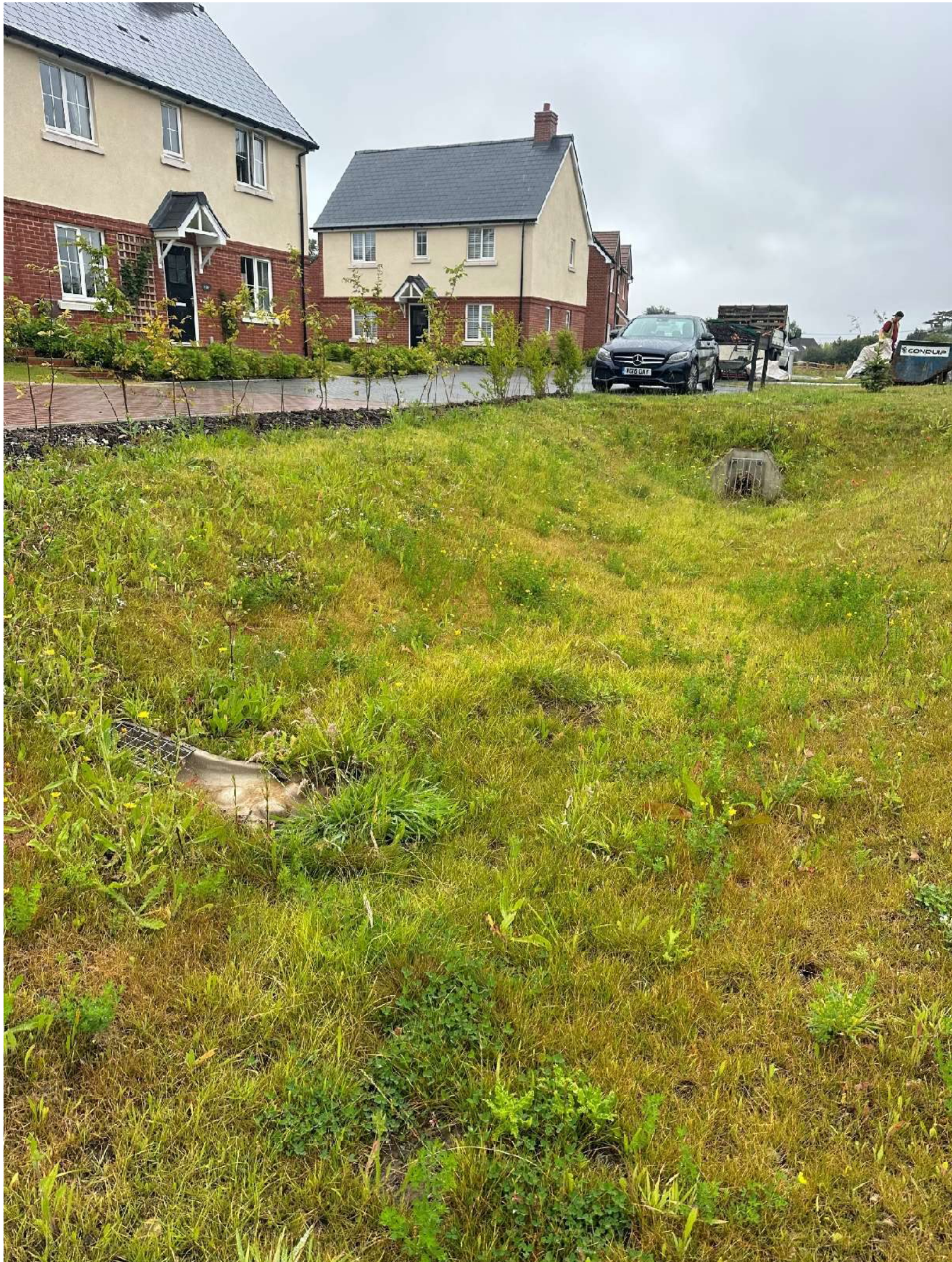
Swale S-HW2F - 9 July 2024 - complete and functioning
