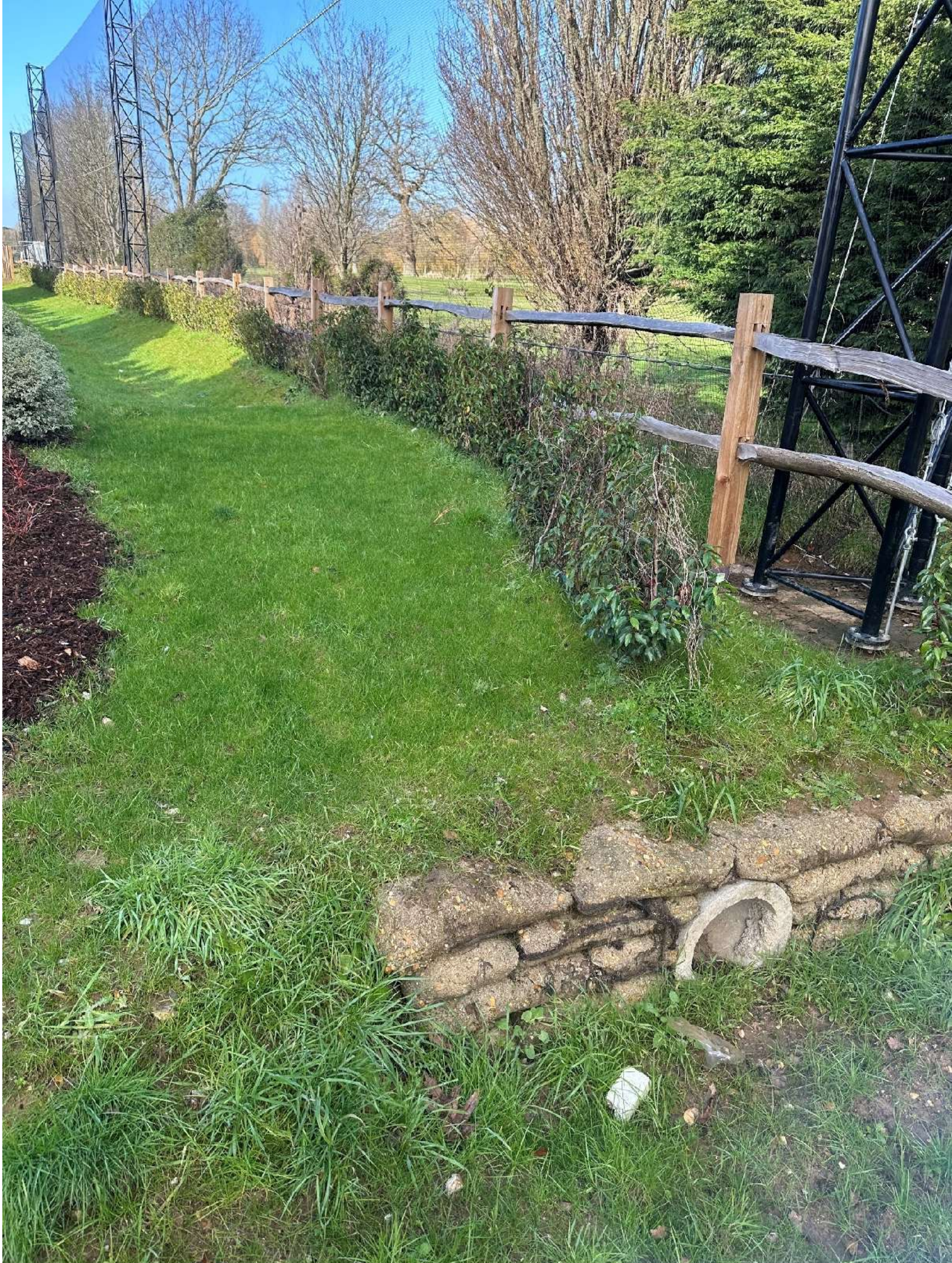
Head Wall 1B - 01 February 2023 - complete and functioning
