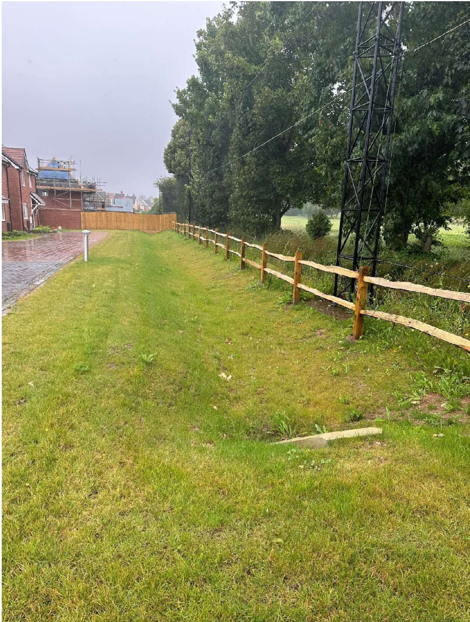
Swale B-HW2A - 9 July 2024 - complete and functioning
