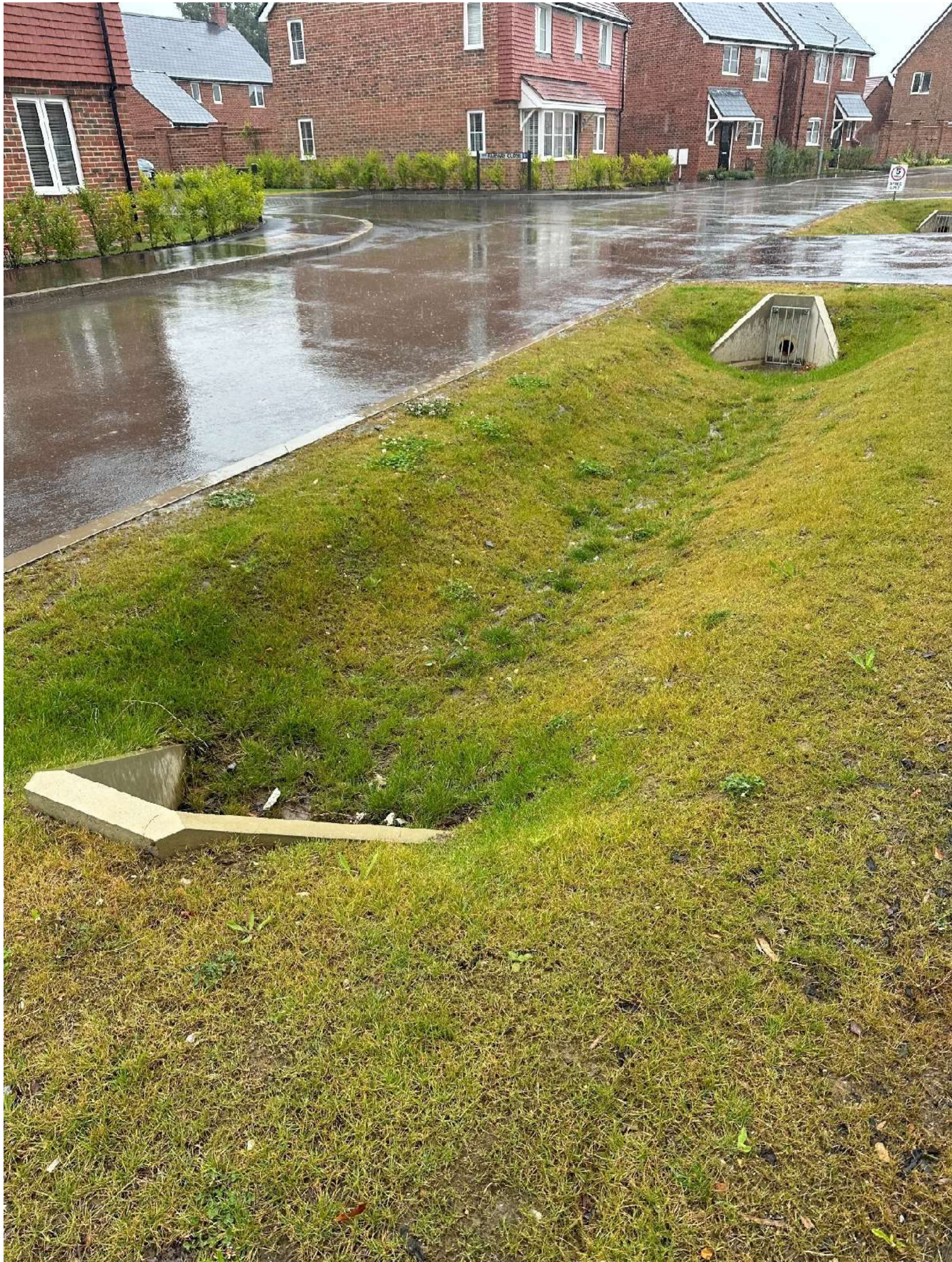
Swale P-Q-HW2C-G - 9 July 2024 - complete and functioning
