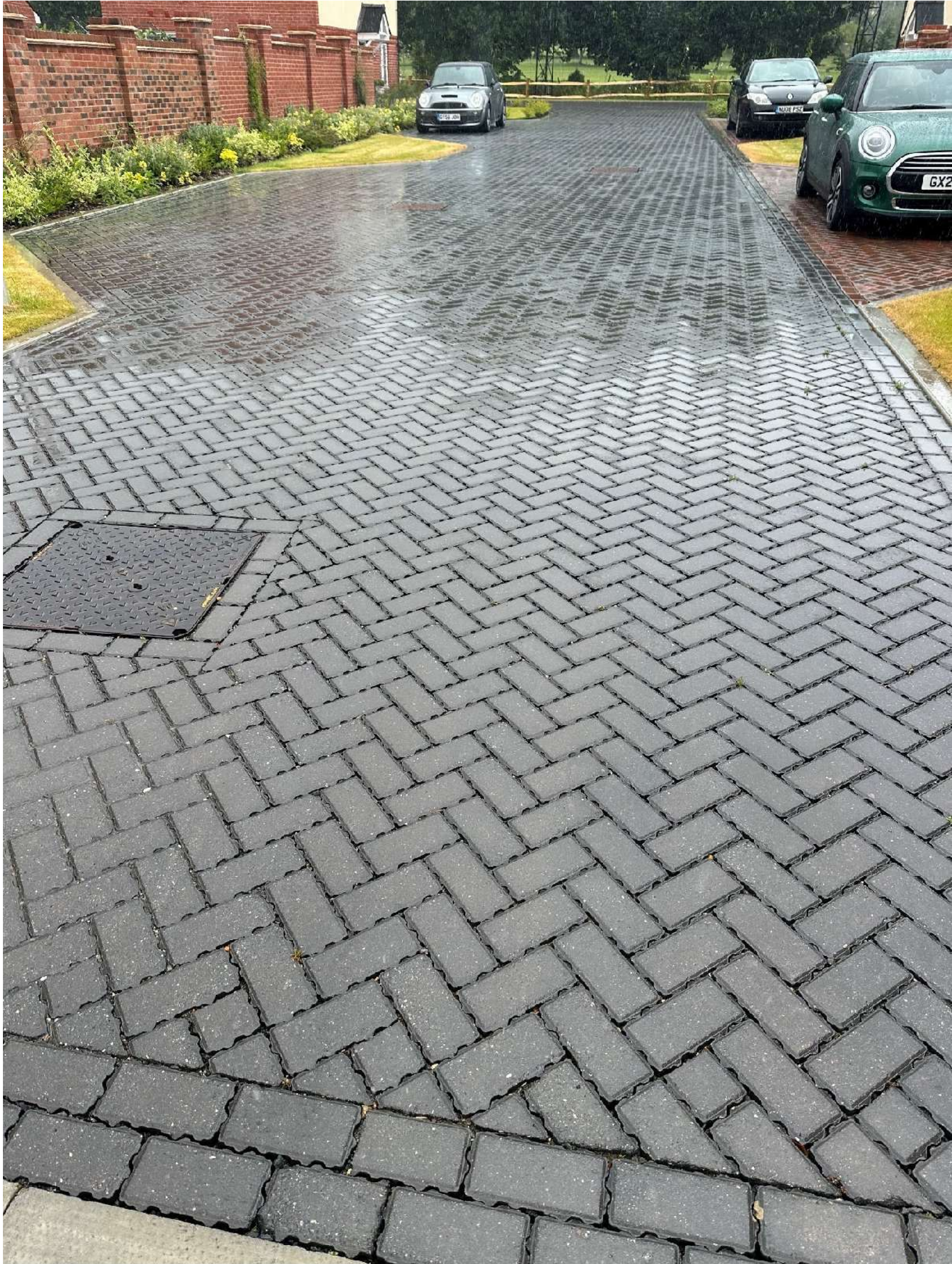
Permeable Pavement 2A - 9 July 2024 - complete and functioning
