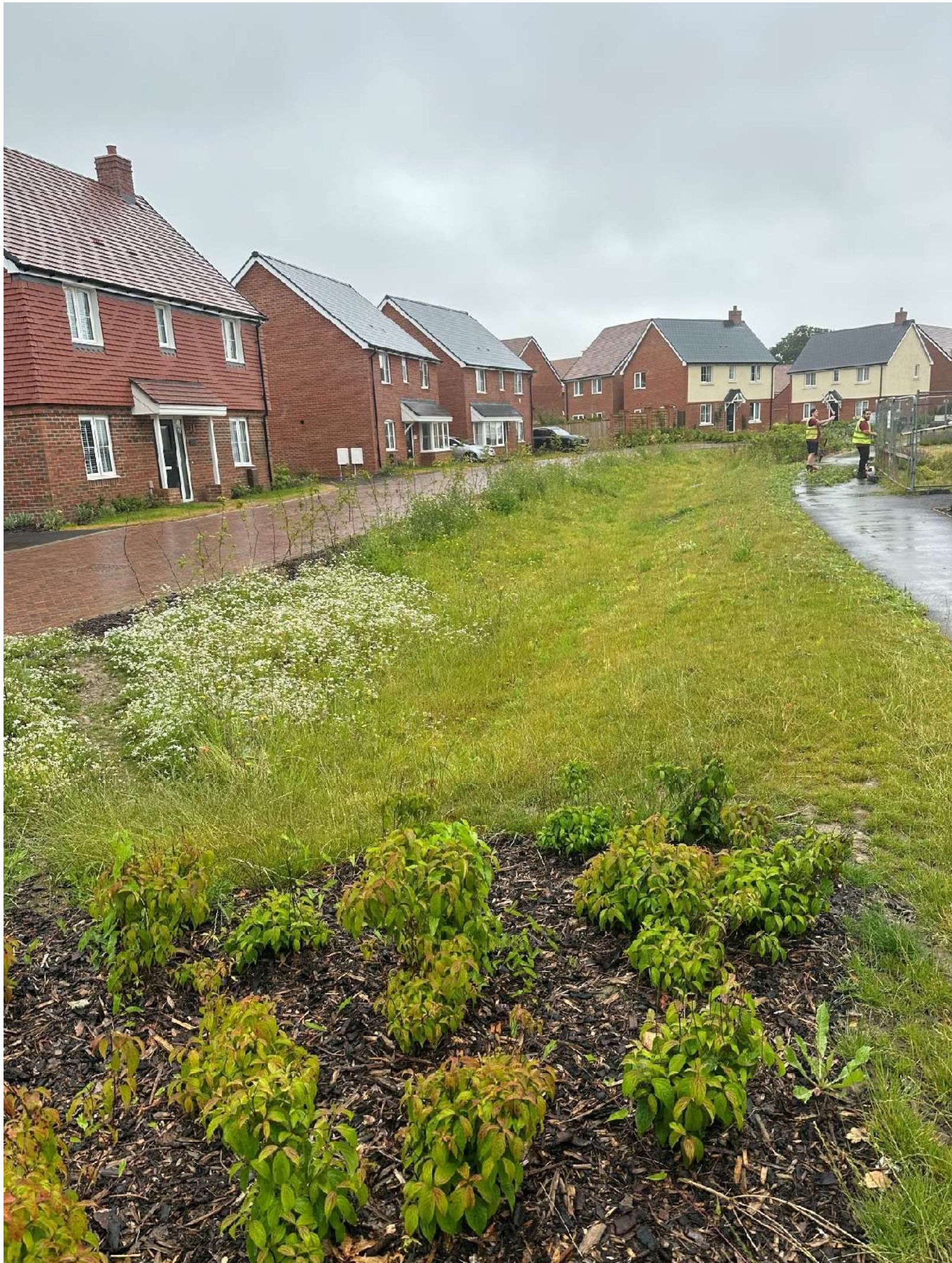
Swale S – 09 July 2024 - complete and functioning
