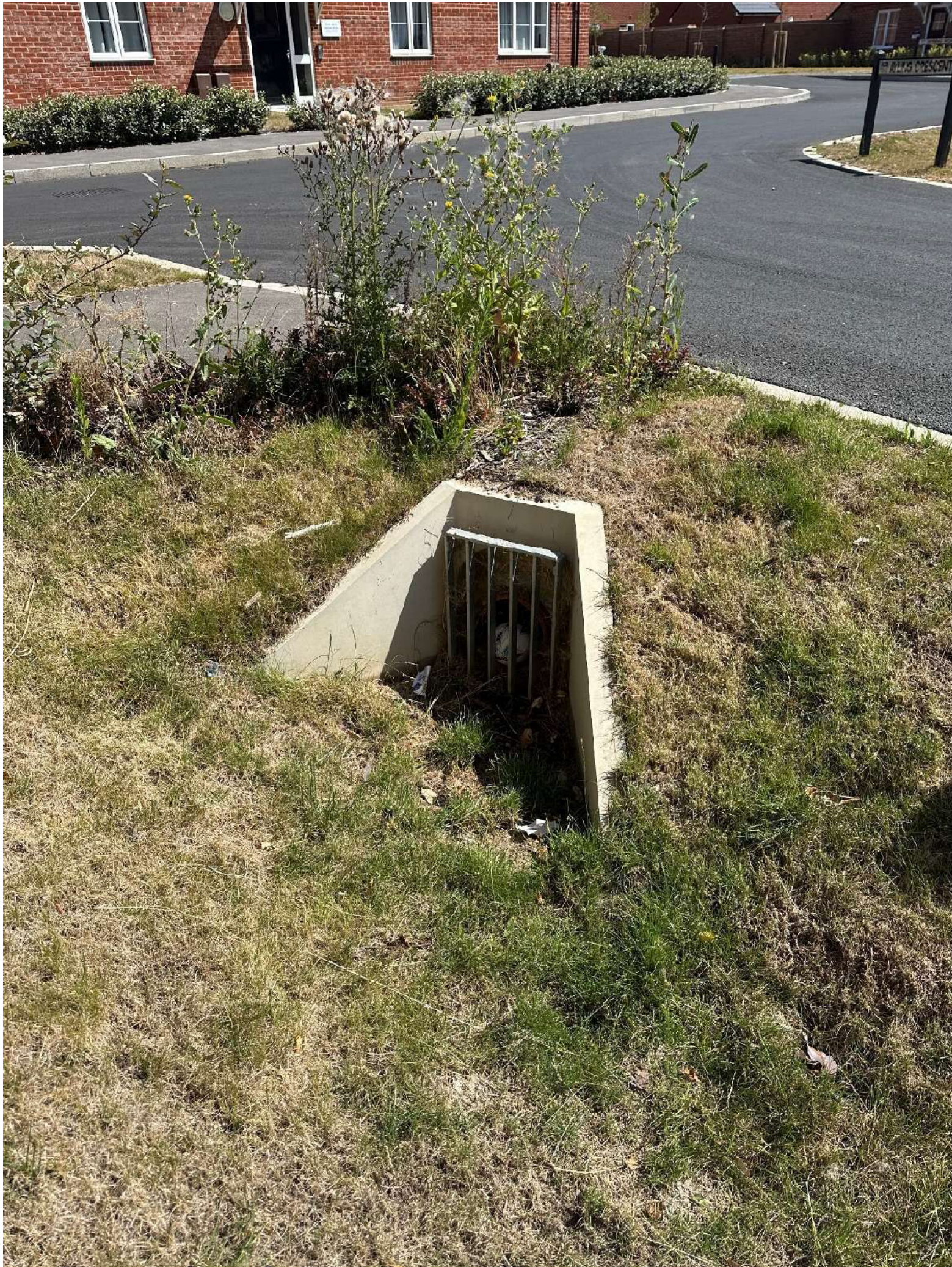
Headwall 3H – 16 th July 2025 - complete and functioning
