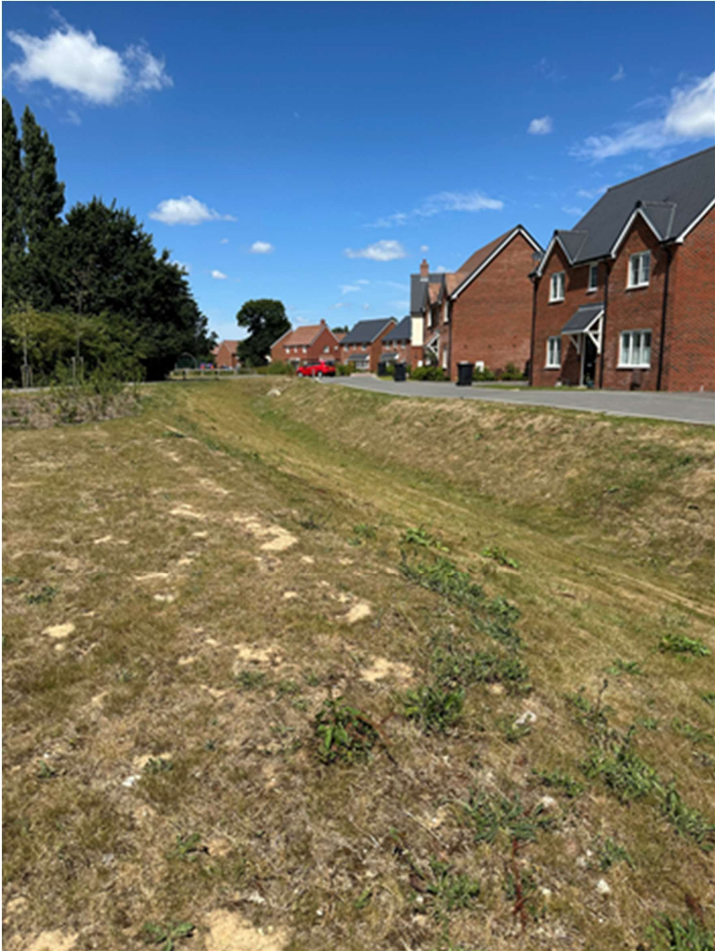
Swale H-HW1F - 16 July 2025 - complete and functioning
