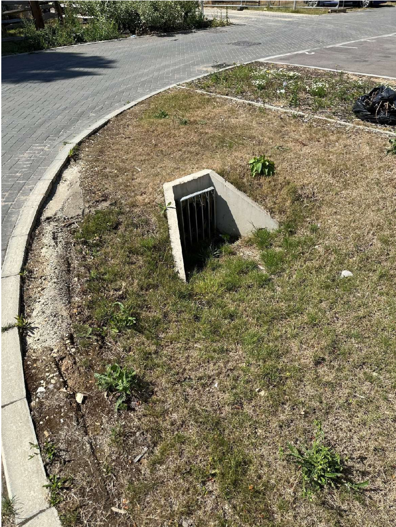
Headwall 3G – 16 th July 2025 - complete and functioning
