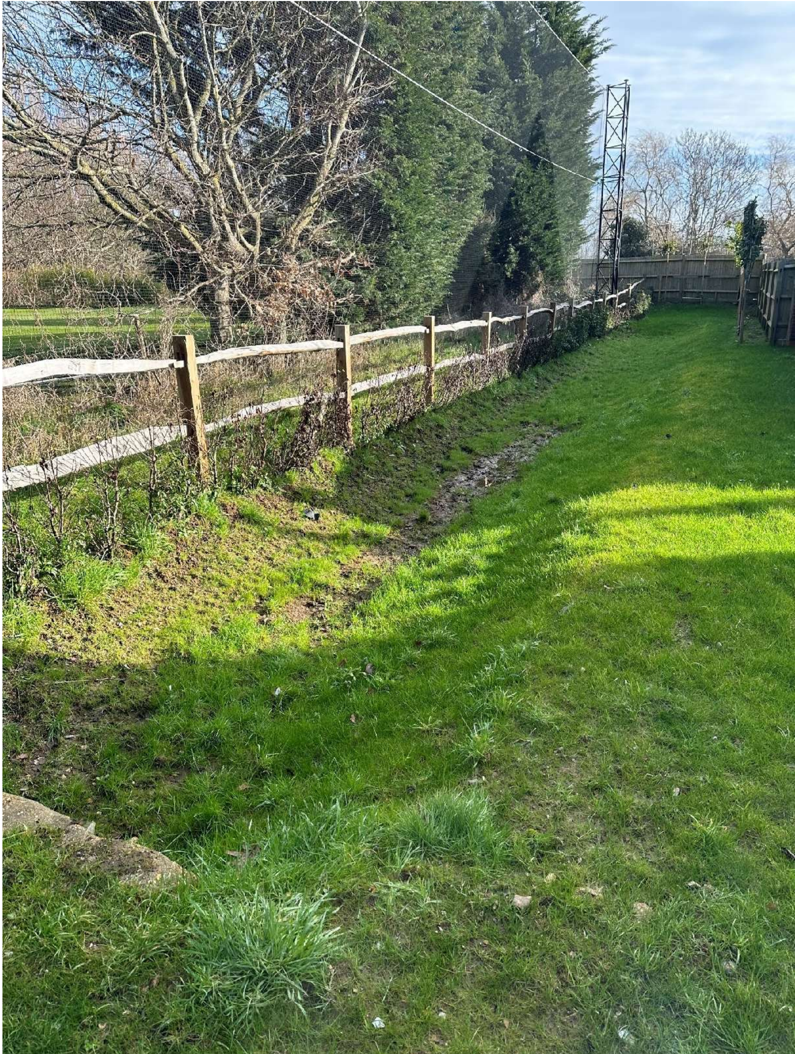
Swale D - 01 February 2023 - complete and functioning
