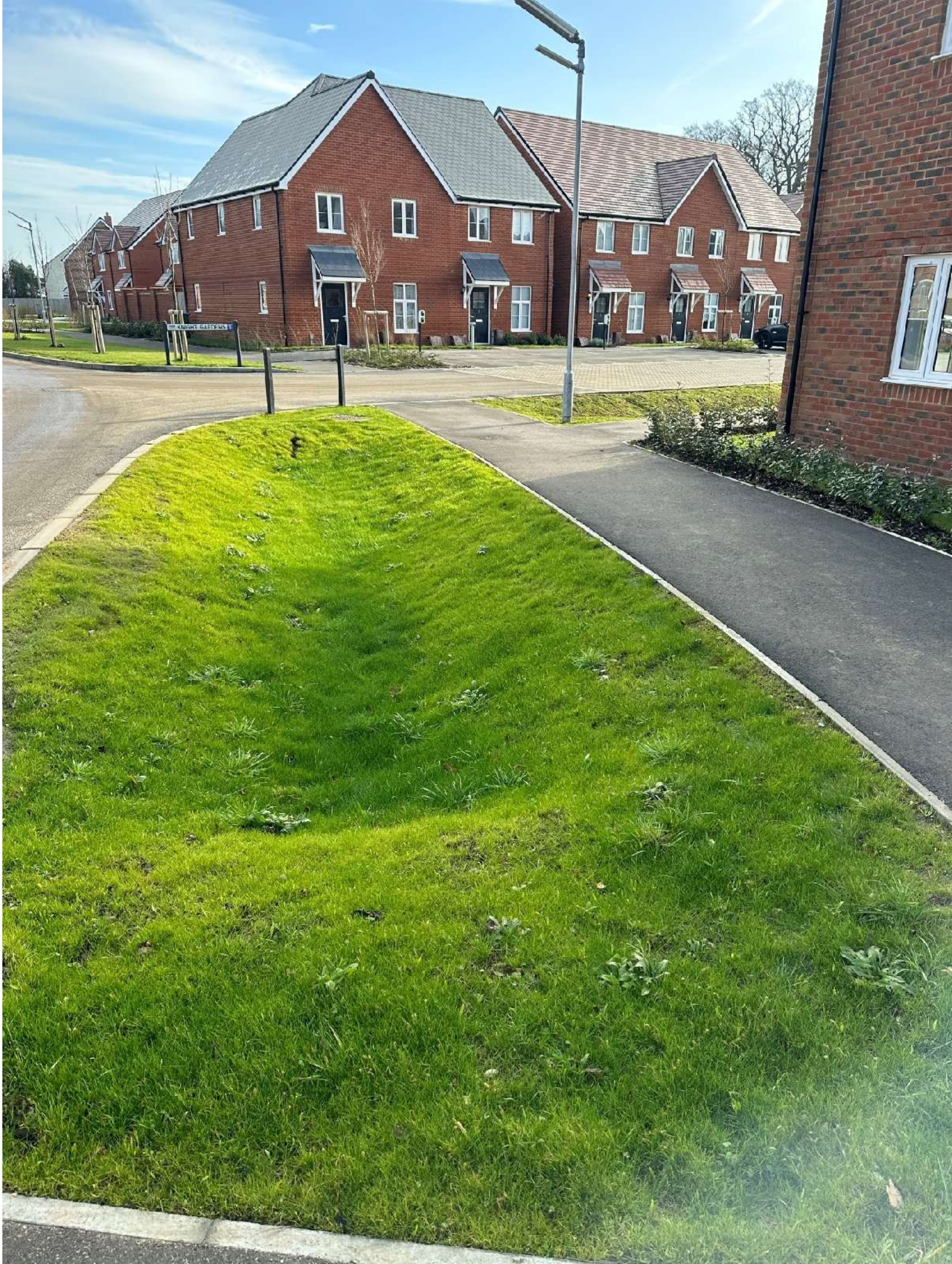
Swale M - - 01 February 2023 - complete and functioning
