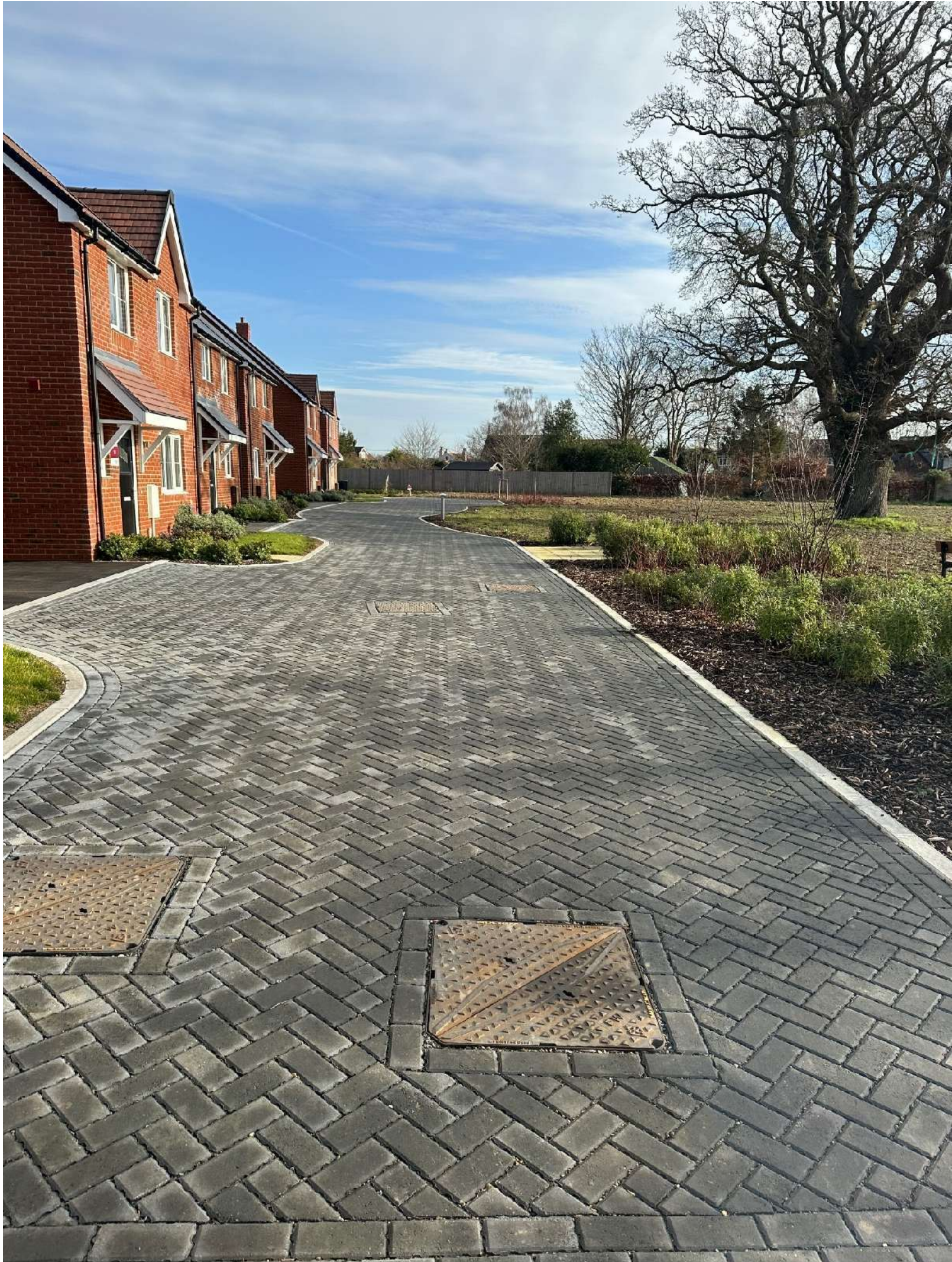
Permeable Paving 1C - 01 February 2023 - complete and functioning
