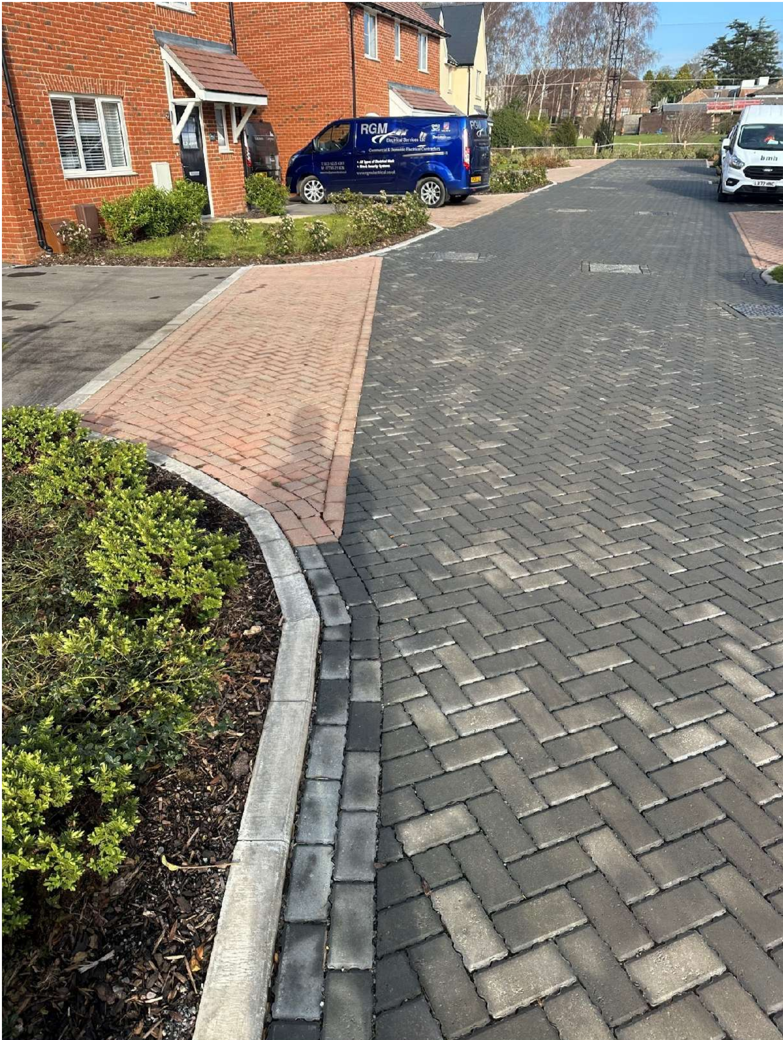
Permeable Paving -1B - 01 February 2023 - complete and functioning
