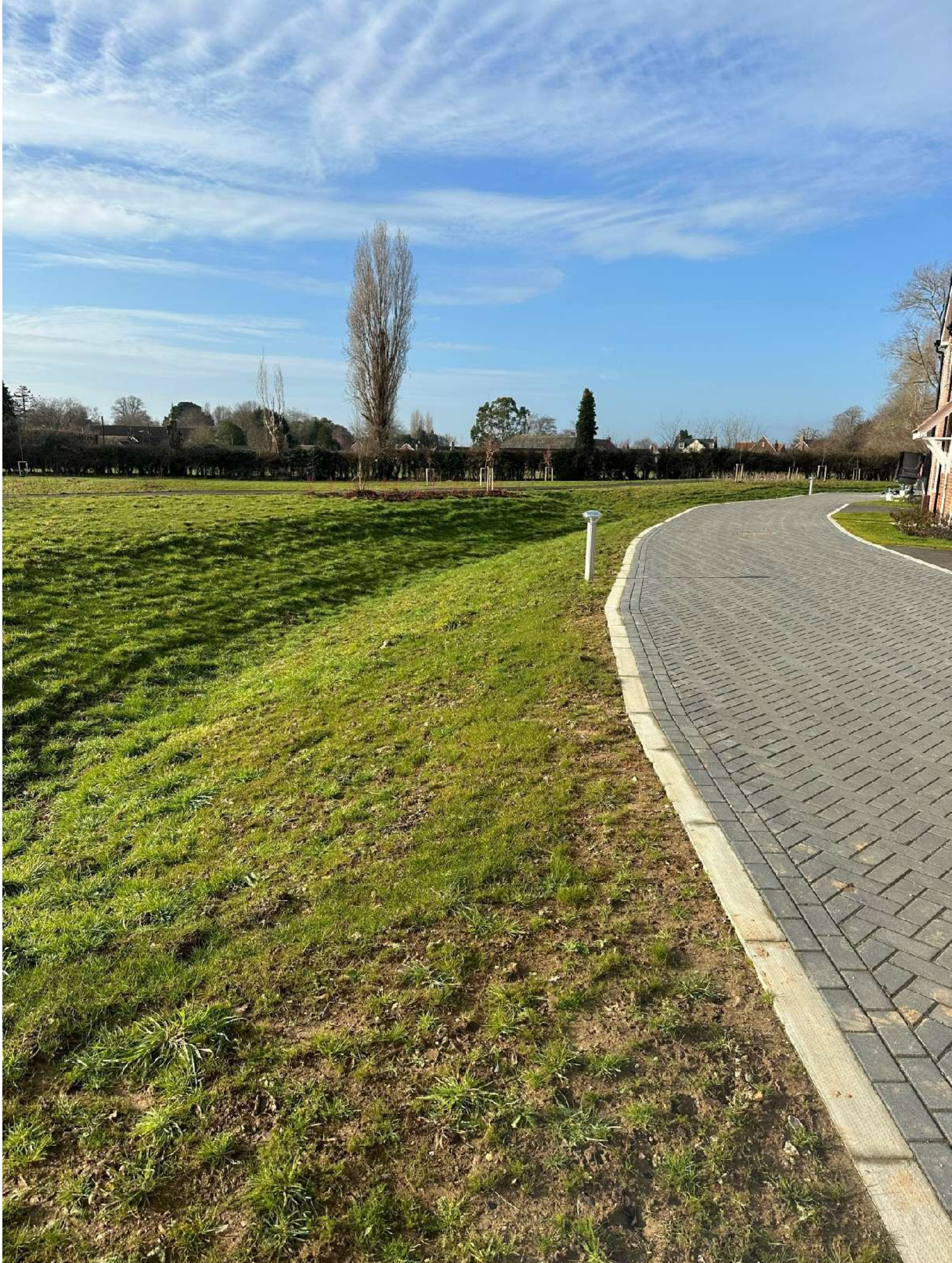
Swale H - 01 February 2023 - complete and functioning
