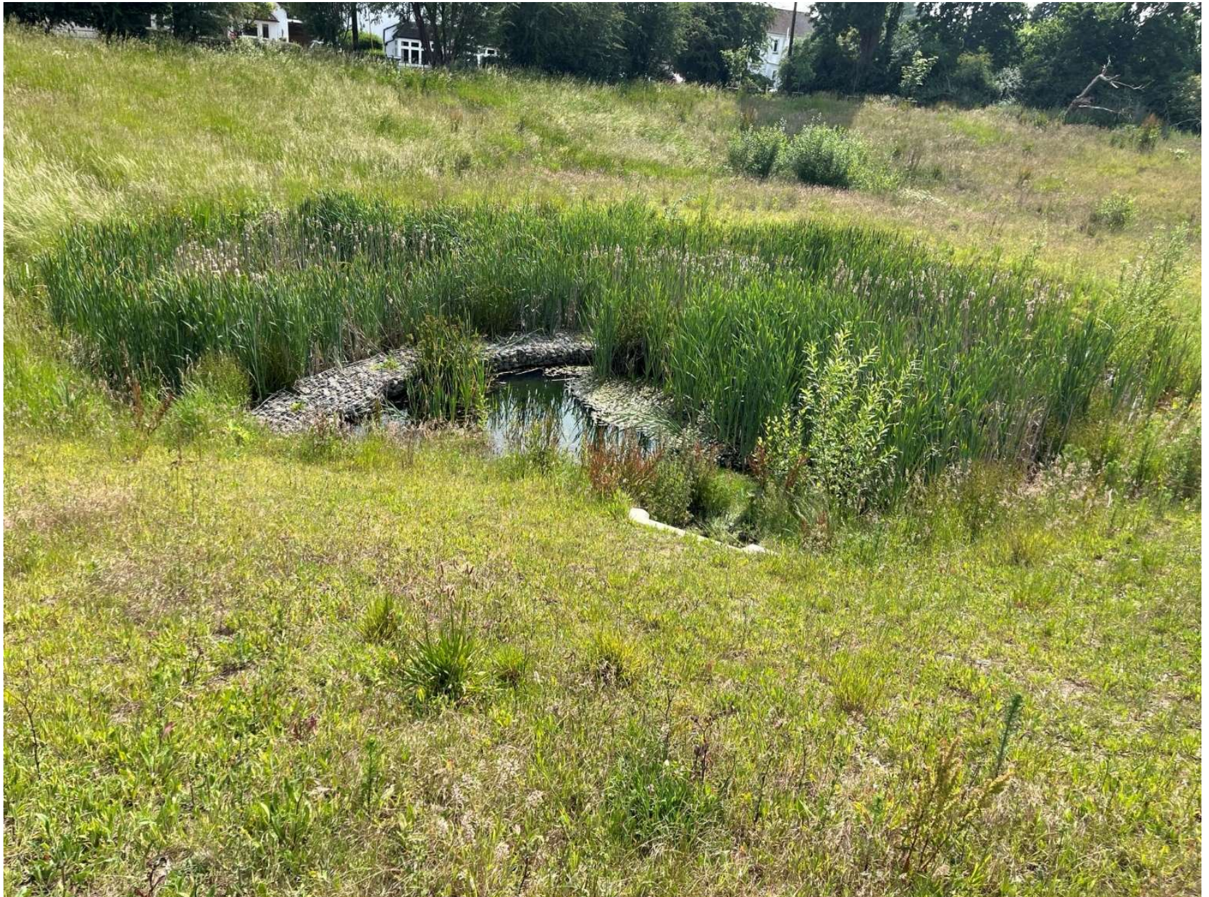
Eastern Pond A - 9 July 2024 - Complete & functioning.
