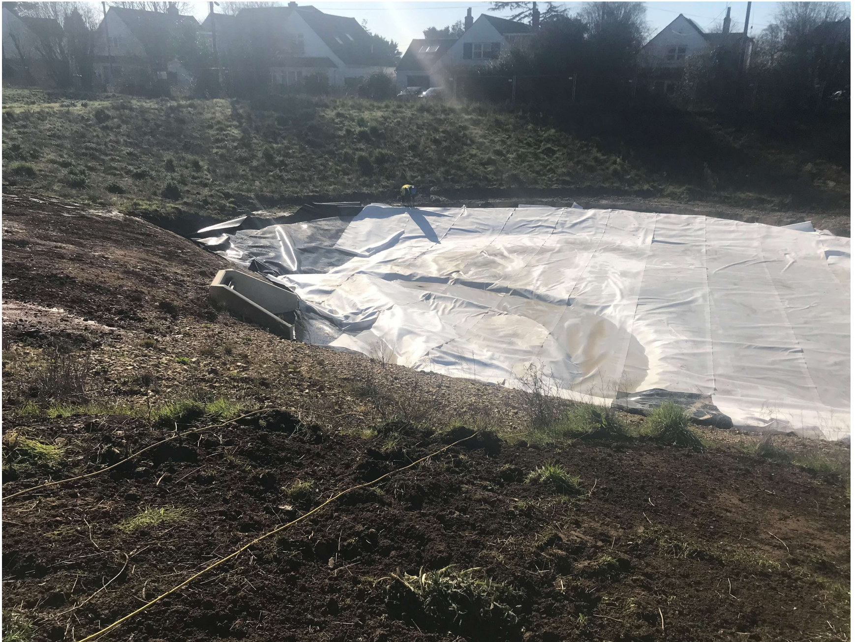
Eastern Pond - 17 March 2022 – under construction, liner being installed.
