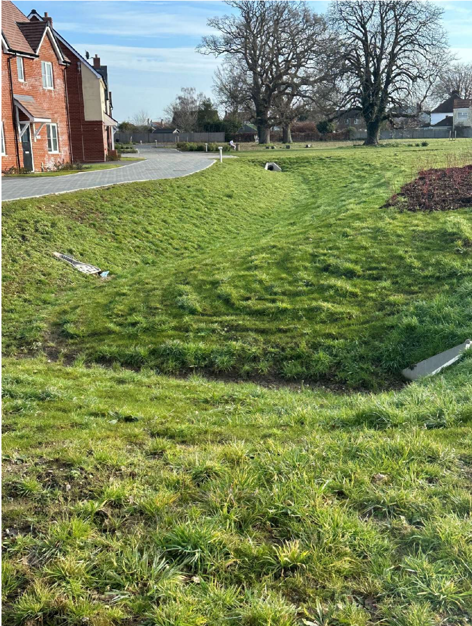
Swale 1H - 01 February 2023 - complete and functioning
