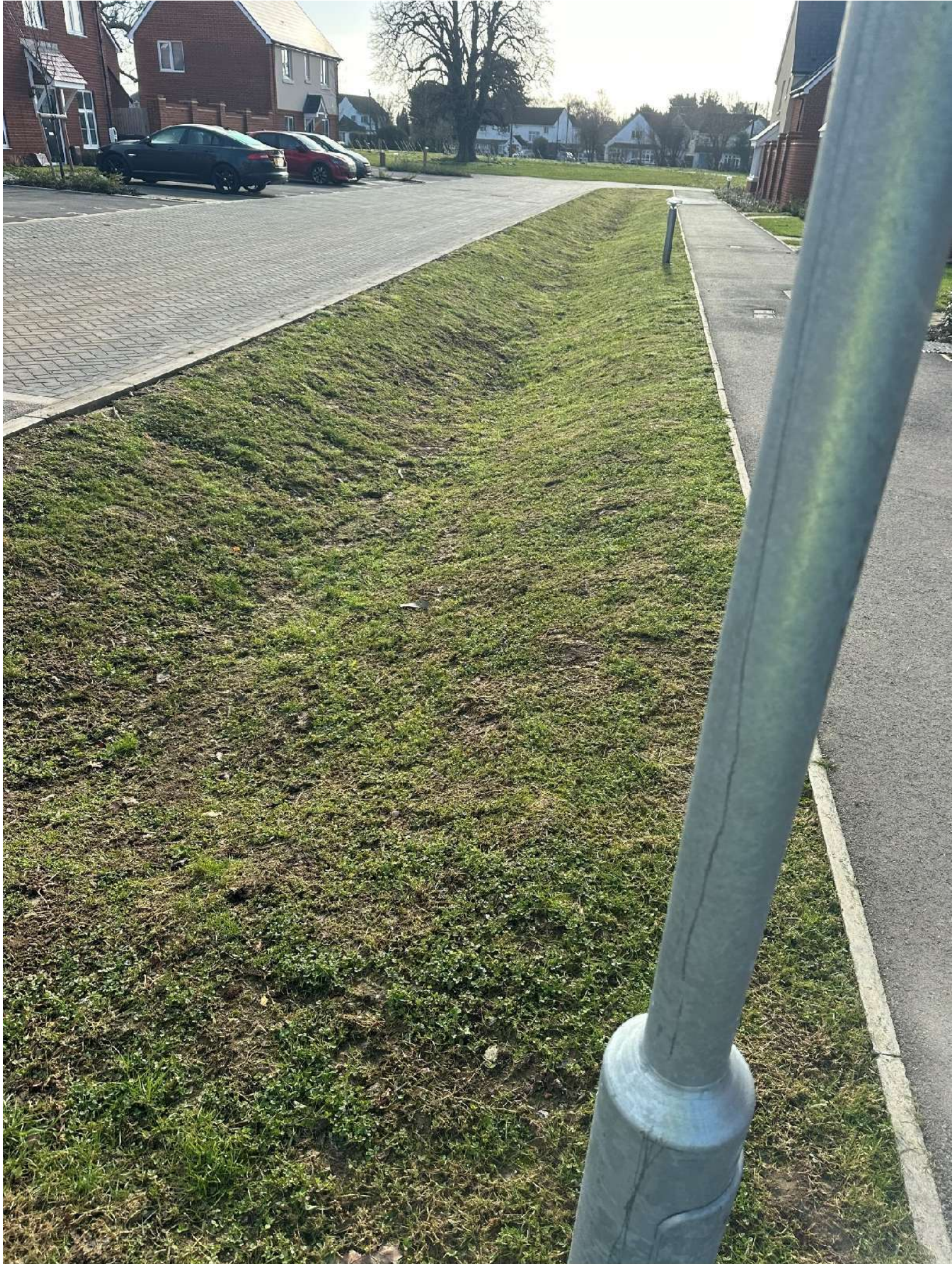
Swale I - 01 February 2023 – complete and functioning
